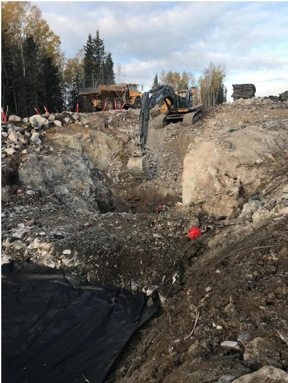
The truck fill building and truck fill pad is one of the last major work items to be completed as part of this CD1 contract. Once the drilling and blasting is completed the piping works will be installed and then the concrete pad poured. As was discussed and approved by the engineer the truck fill building drain will be realigned and installed in the common trench with the water main servicing the building this will eliminate the need for a second trench being blasted.
