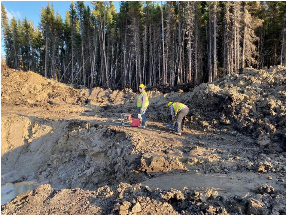
In preparation for the drilling and blasting for the balance of the onsite piping and onsite liftstation the trenches have been stripped of overburden and sloped to allow safe access for the drills and sewer and water crews.
