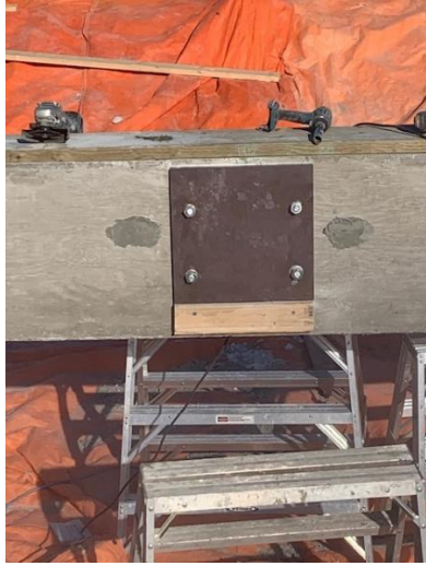
Steel plate installation on Center Beam
