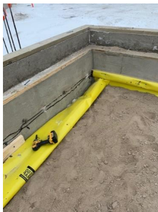
Poly Installation and sand in Crawlspace
