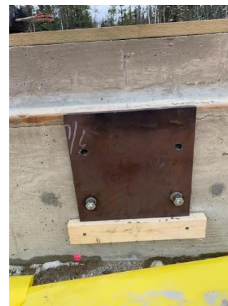
Steel plate installation on Grade Beam
