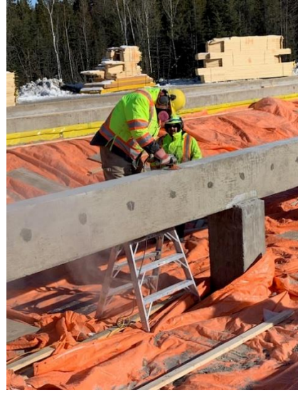
Grind and Levelling Center Beam
