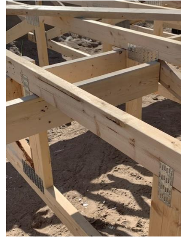
Strong Back Installation for Floor Joist
