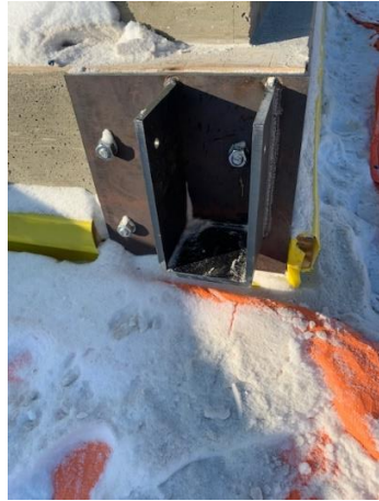
Welded Steel Saddle Installation
