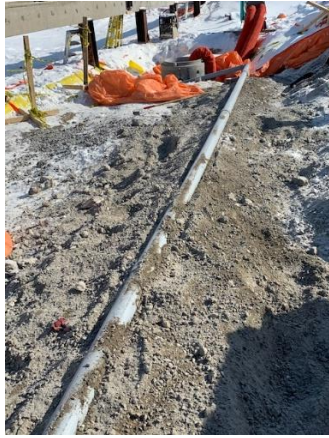
Drainpipe from Elevator Pit to Sump Pit Installation
