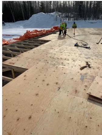
Main Floor Sheathing Installation
