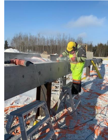
Grind Down Center Beam
