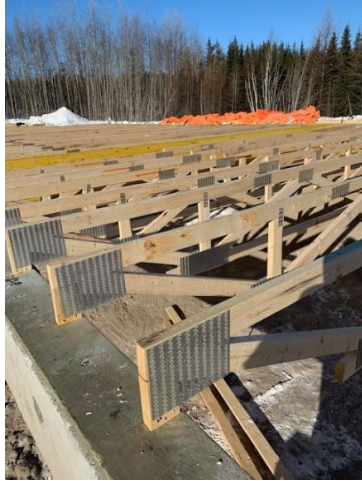
Floor Joist Installation
