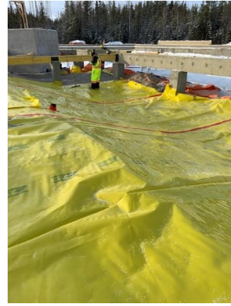
Poly Installation in Crawlspace
