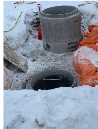
Riser Install on Sump Pit
