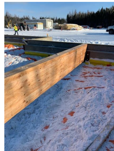
Installation of Wood Beams
