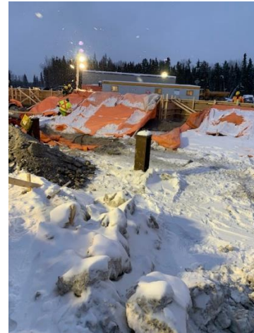
Remove hoarding and formwork from grade beam
