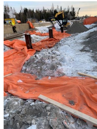
Ground thaw for weeping tile trench
