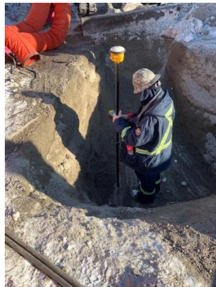
Verify depth of sump pit
