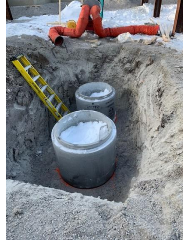
Sump pit base placement
