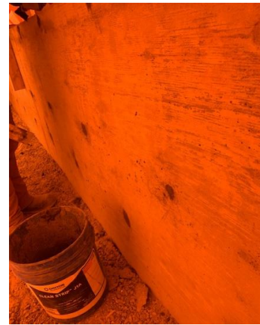
Grout tie holes in grade beam
