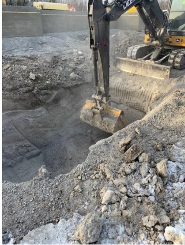
Excavating for sump pit
