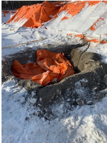
Ground thaw for sump pit excavation
