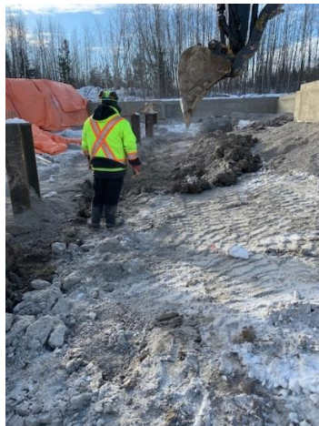
Excavating weeping tile trench
