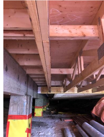
Poly Installation on Concrete Piers
