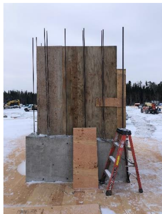
Elevator Shaft Formwork
