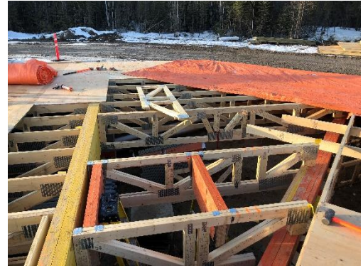
Floor Truss Installation
