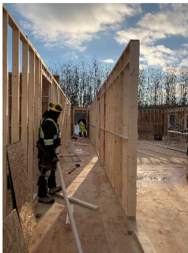
Corridor Wall Framing
