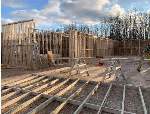
Interior Wall Framing
