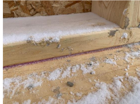
Sill Gasket Installation
