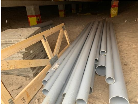
Staging Mechanical Material in Crawlspace
