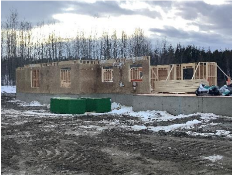
Prefab Exterior Wall Installation
