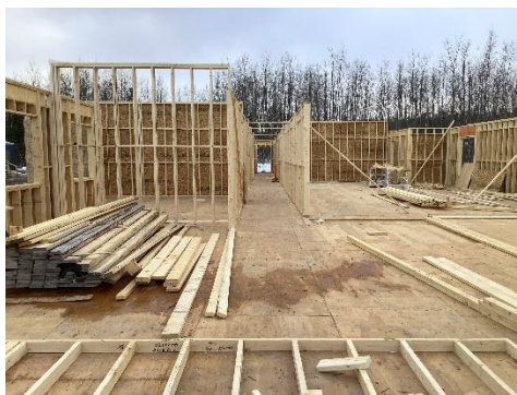
Interior Wall Framing
