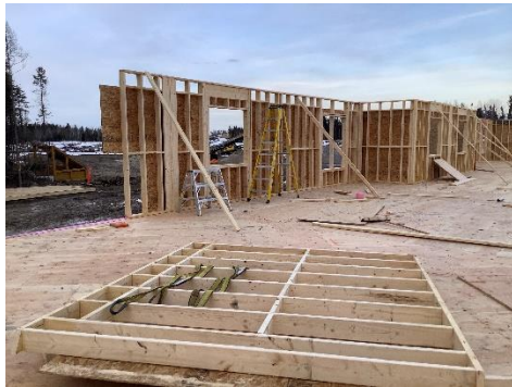
Exterior Wall Framing
