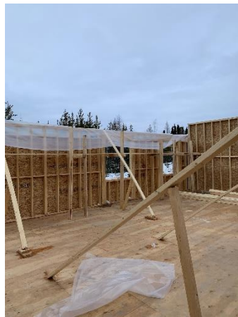
Vapour Barrier Installation
