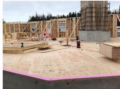
Sill Gasket Installation
