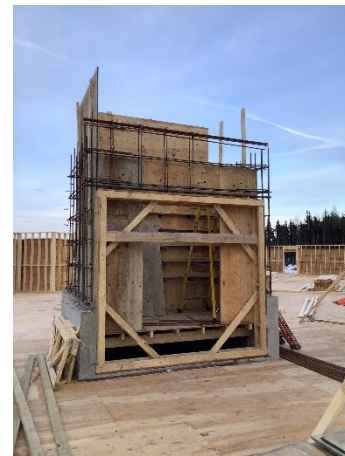
Elevator Shaft Wall Rebar
