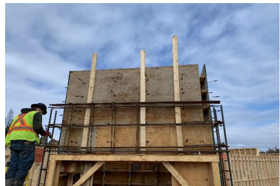
Elevator Shaft Wall Rebar Install
