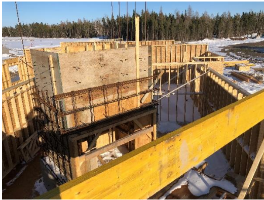
Second floor LVL Install
