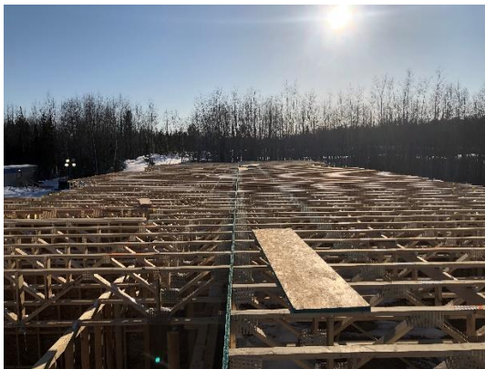
Second Floor Wood Truss Install
