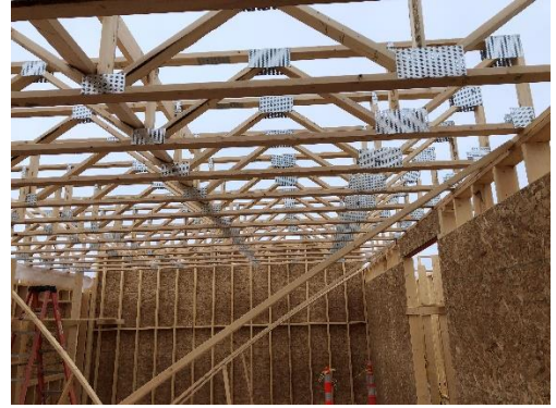
Second Floor Wood Truss Install
