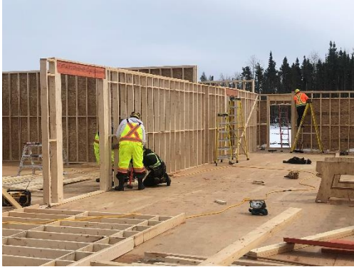
Interior Wall Framing
