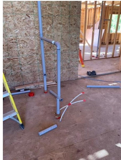
Plumbing Lines Install on Second Floor – West Wing
