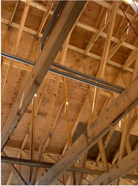
Electrical Conduit Install in Attic Space – West Wing
