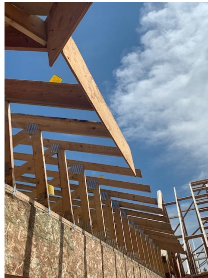
Fascia Board Install – West Wing
