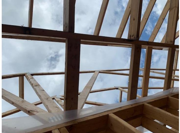
Roof Blocking Install – East Wing
