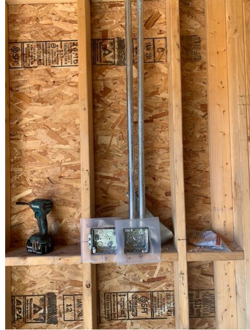
Electrical Boxes Install on Main Floor – East Wing
