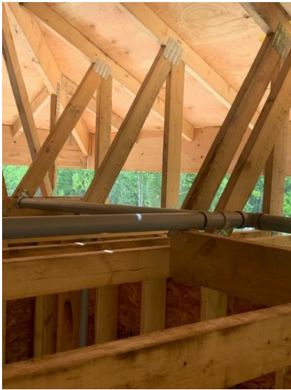
Plumbing Vent Lines Install in Attic Space
