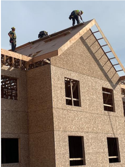
Roof Sheathing on Gable End – West Wing
