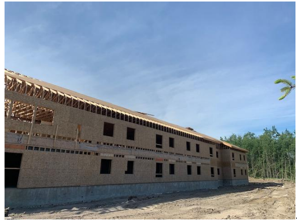
Exterior View – North West Side
