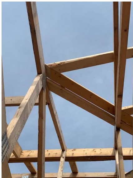
Roof Framing Install – North Side
