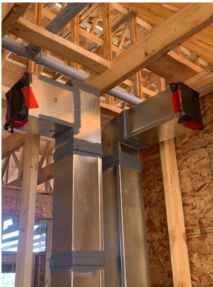
Duct Work Install on Second Floor – West Wing
