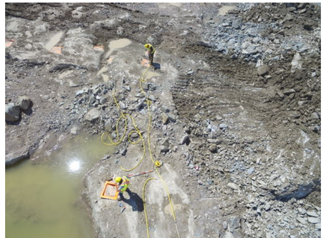
Drilling for pad locations
