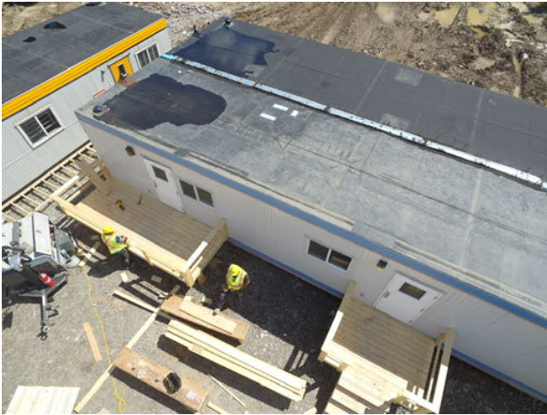
Trailer deck railing framing
