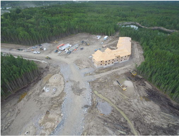
Site access road towards P.A project Wayne Dee Jul 17, 2020 3:28 PM
