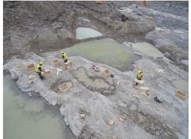
Concrete pad form work framing Wayne Dee Jul 17, 2020 3:28 PM
