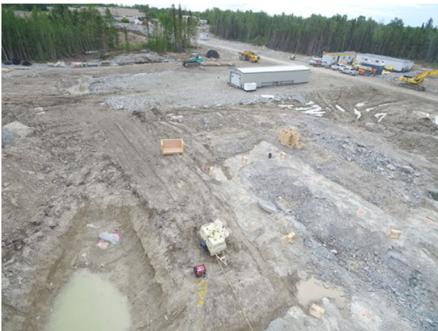
Drone shot of site office setup Wayne Dee Jul 17, 2020 3:28 PM
