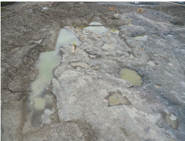
Concrete pad form work framing Wayne Dee Jul 17, 2020 3:28 PM
