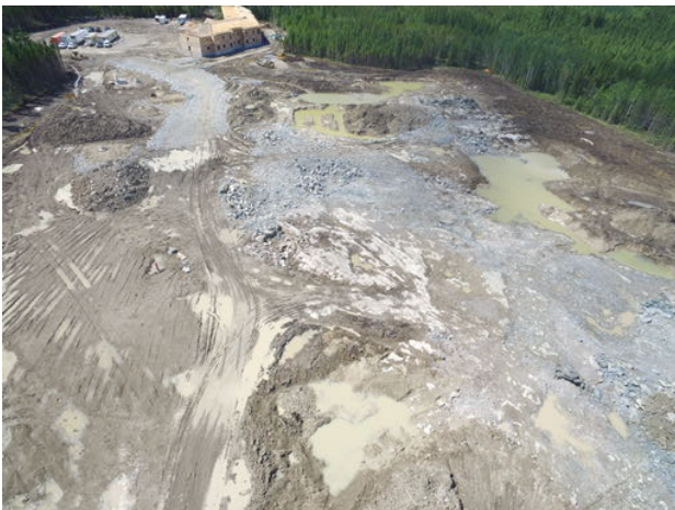
Preparation for dewatering due to heavy rainfall
