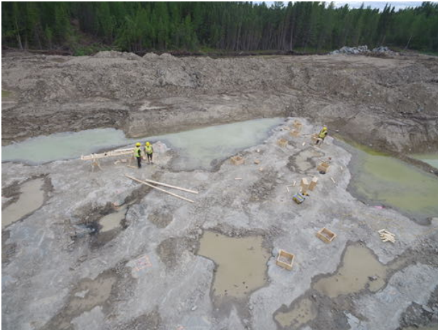
Concrete pad form work framing
