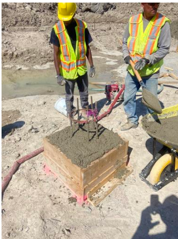
concrete placing in pad location Wayne Dee Aug 7, 2020 3:31 PM
