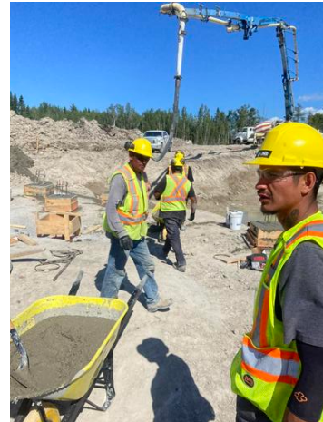
Concrete pump line Wayne Dee Aug 7, 2020 3:31 PM
