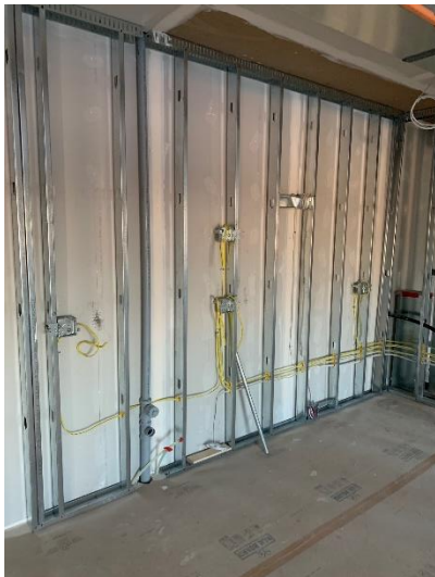
Electrical Box and Wiring Install On Second Floor Suite - East Wing
