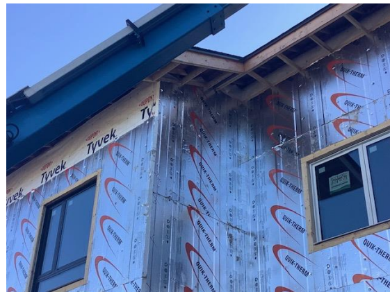
Exterior Rigid Insulation Installation - South East Wing
