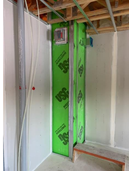
Mechanical Chase Enclosed on Second Floor Suite – West Wing
