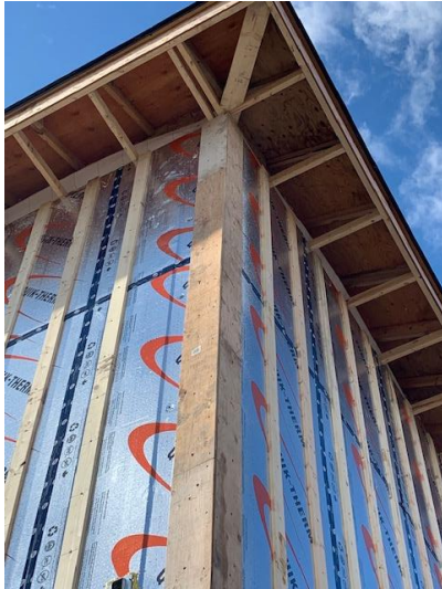
Exterior Strapping Install – North East Wing
