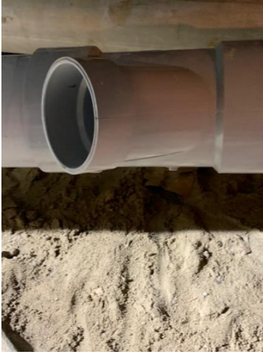
Sanitary Line Install in Crawlspace
