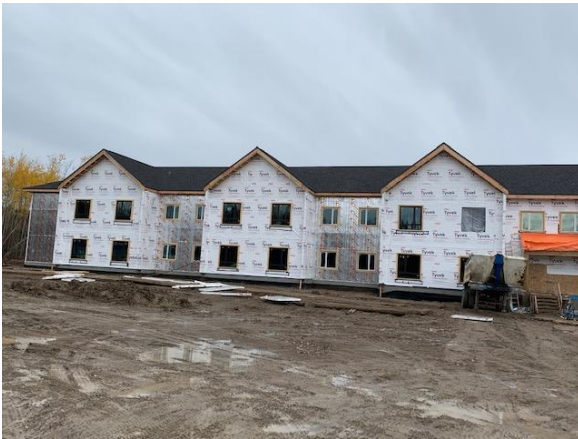
Exterior View – South West Wing
