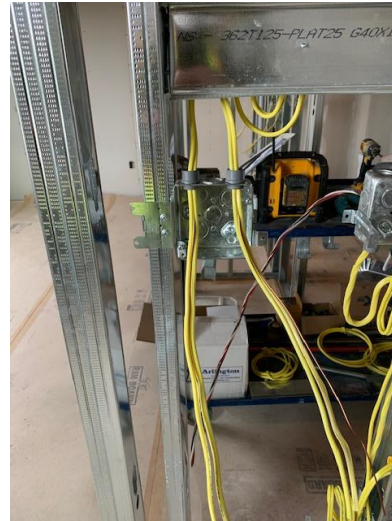
Electrical Wiring Pull on Second Floor Suite – West Wing
