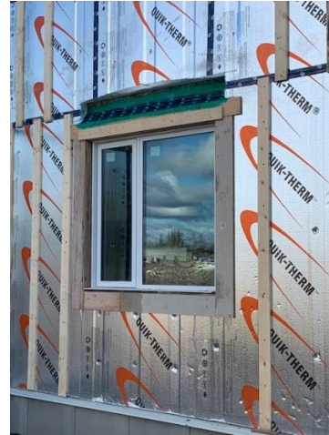
Above Window Blueskin and Flashing Install – North East Wing
