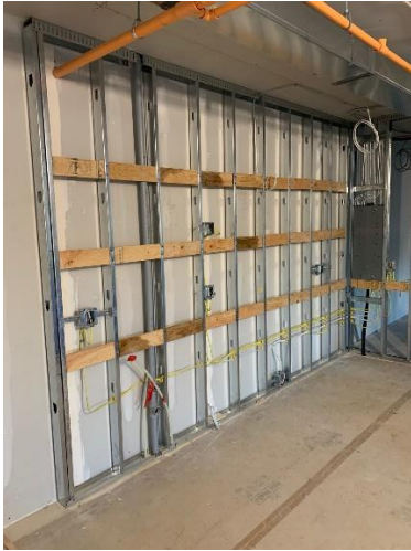
Wood Backing Install in Steel Stud Walls on Second Floor
