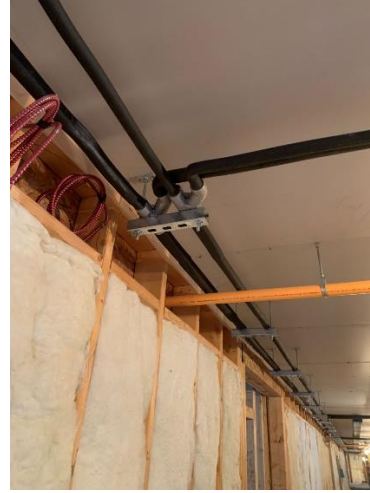
Refrigeration Line with Insulation Install on Second Floor Corridor – West Wing
