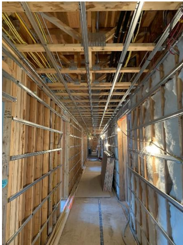
Resilient Channel Install On Main Floor -Ceiling and Wall - East Wing
