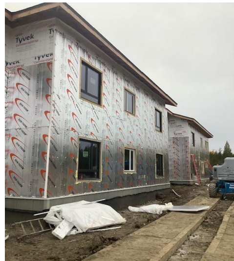
Exterior View – North East Wing
