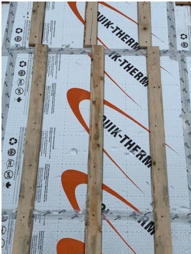
Exterior Strapping Install - South West Wing
