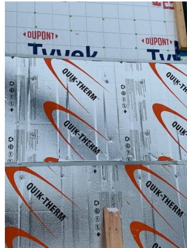
Exterior Rigid Insulation Install - South West Wing
