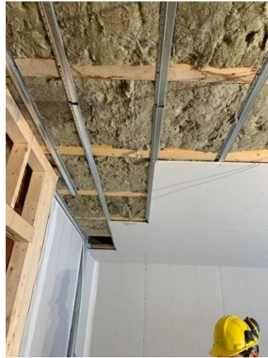
Gypsum Board Install on Main Floor Ceiling – East Wing
