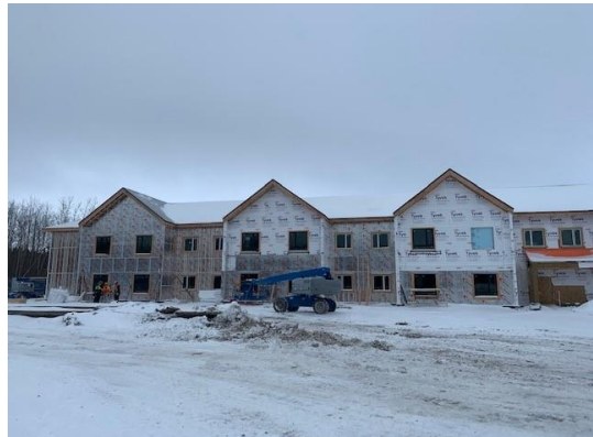
Exterior View – South West Wing
