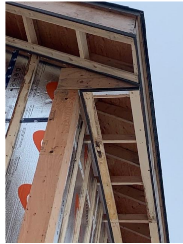
Soffit Framing – North West Wing
