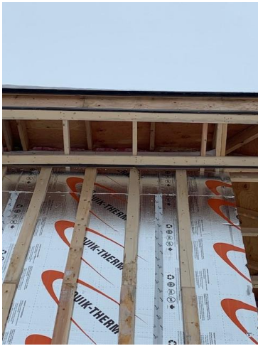
Soffit Framing – North West End
