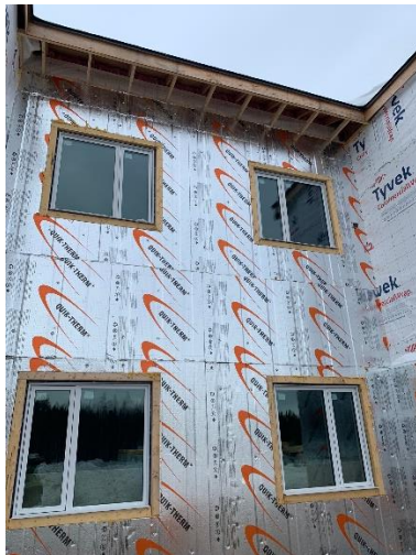
Exterior Rigid Insulation Install – South East Wing
