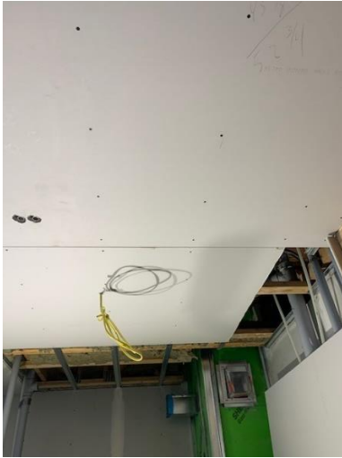
Gypsum Board Install on Main Floor Ceiling – West Wing
