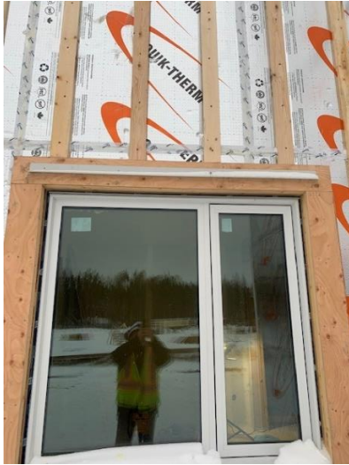
Window Head Flashing Install Lower Level – South West Wing
