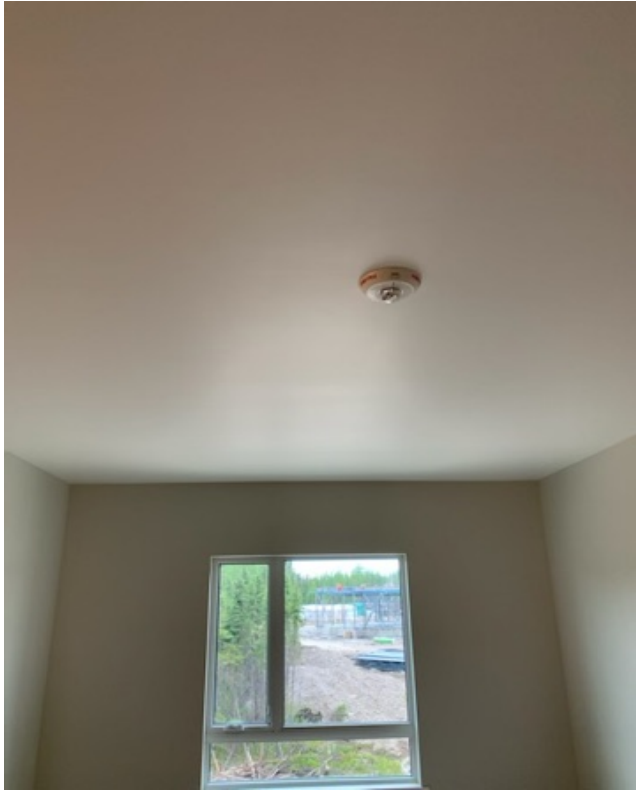
LVL 2 EW Ceiling Final Paint
