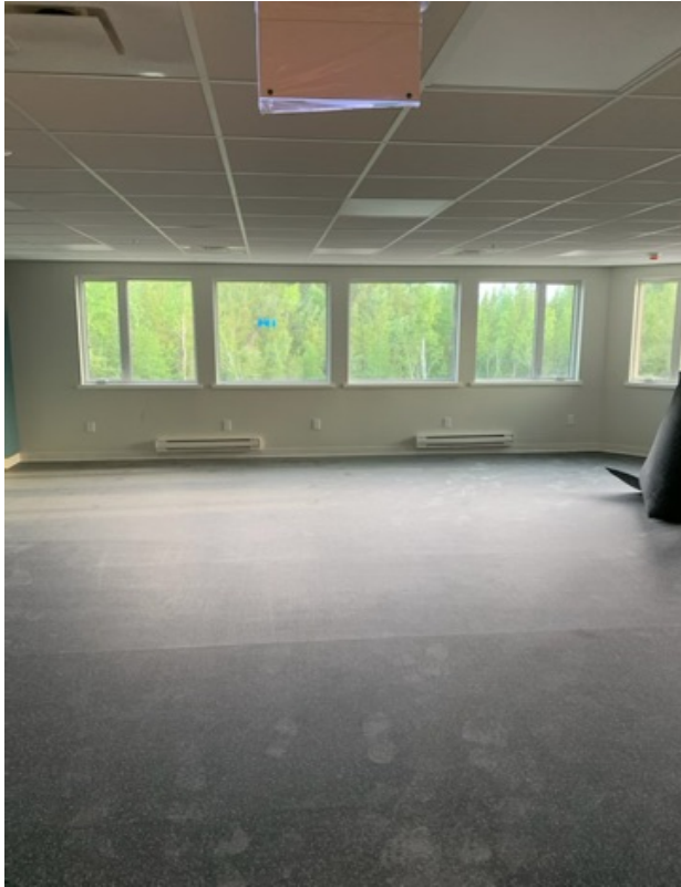
LVL 2 Fitness Centre Progress
