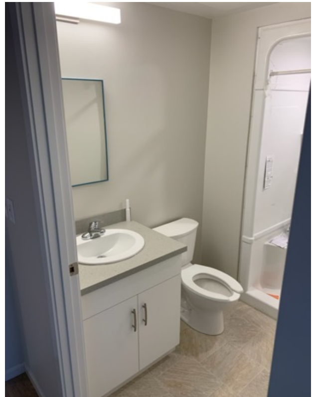
LVL 2 EW Suite Washroom Progress
