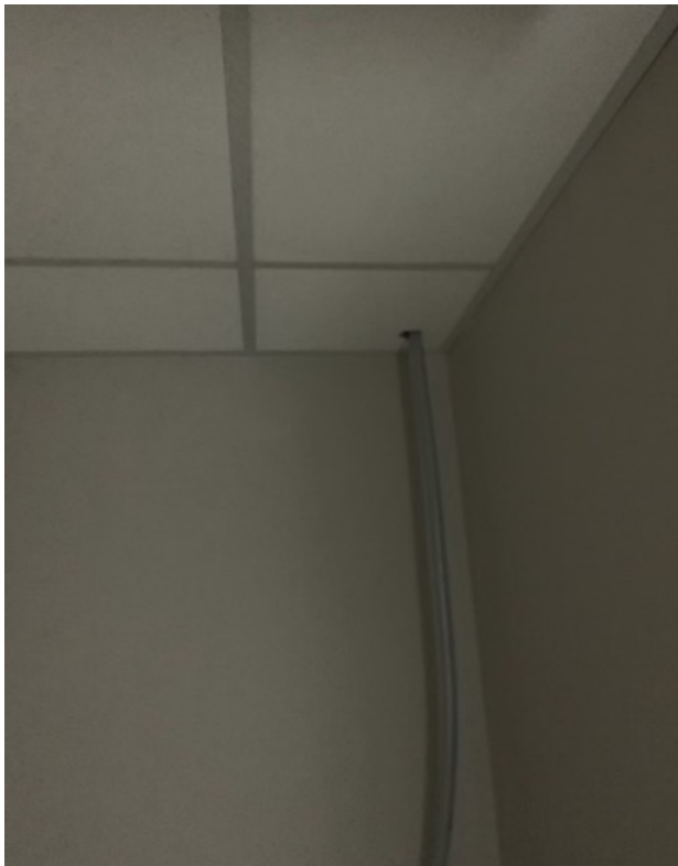
ACT cut to accommodate condensate piping
