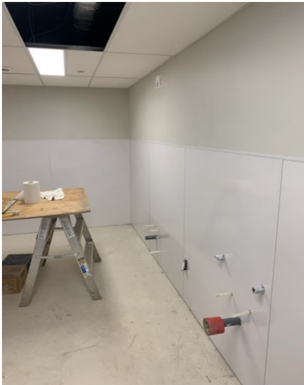
LVL 1 Laundry Room FRP Install
