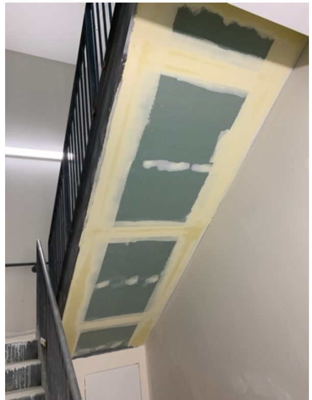
Stair 3 Taping Progress
