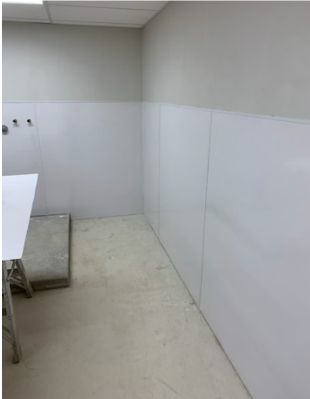
LVL 1 Laundry Room FRP Install
