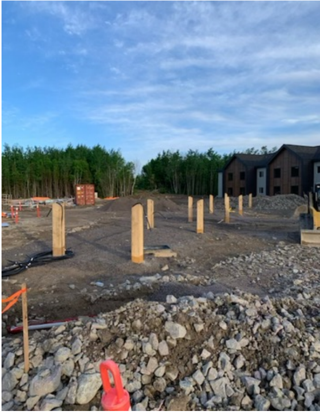
Exterior Parking Outlet Post Install
