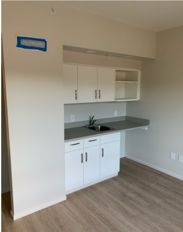
LVL 2 WW Suite Progress
