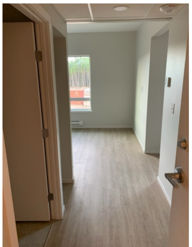
LVL 2 WW Suite Progress
