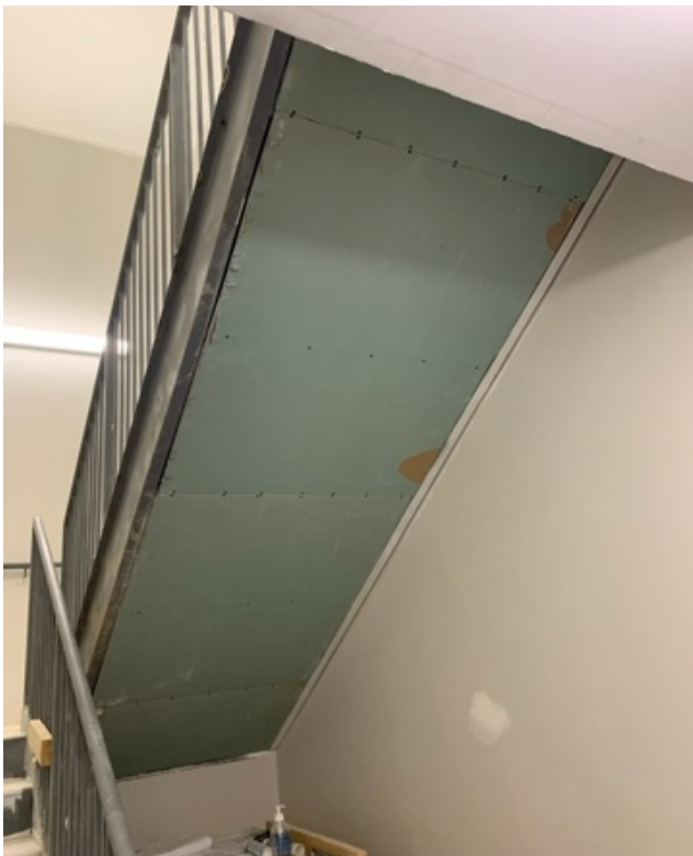
Stair 3 Boarding Progress
