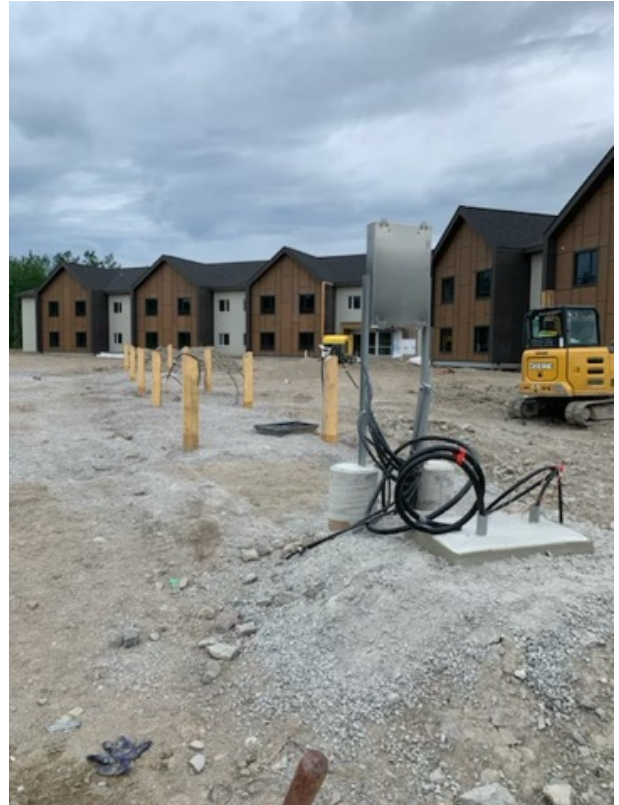
Exterior Parking Lot Panel/Transformer Install
