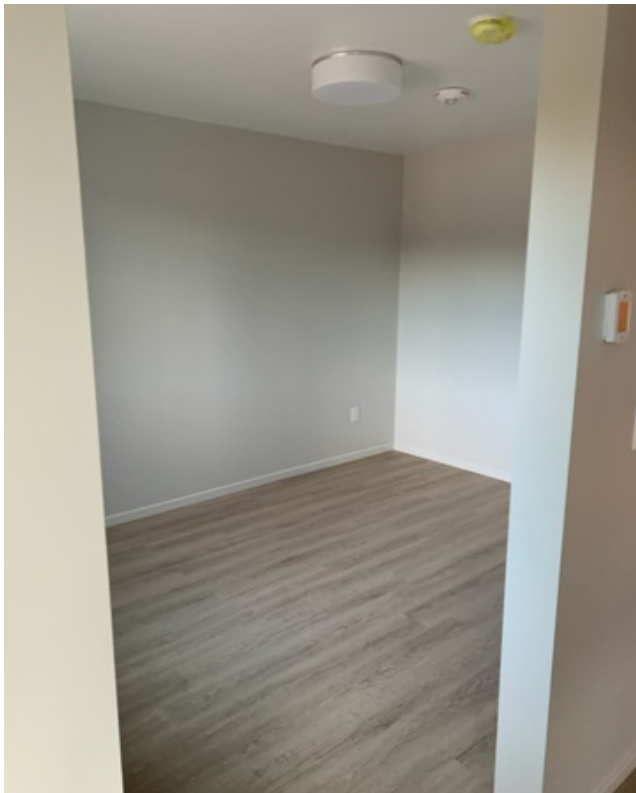
LVL 2 WW Suite Progress
