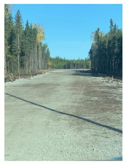
Near the new professional accommodations in the area where the new parking lots are to be established rock fill has been hauled in to create a rock laydown pad for the construction activities. This area will be later brought up to final grate with a combination of 4" material and traffic gravel and then paved at the completion of the project. For the construction period it is the intention to leave it as a gravel pad.
