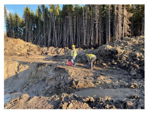
In preparation for the drilling and blasting for the balance of the onsite piping and onsite liftstation the trenches have been stripped of overburden and sloped to allow safe access for the drills and sewer and water crews.
