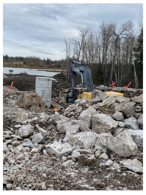
The drilling and blasting continued towards the road crossing to complete the drilling and blasting of the high rock that was located between the lift station and the road crossing which was drilled and blasted last week.
