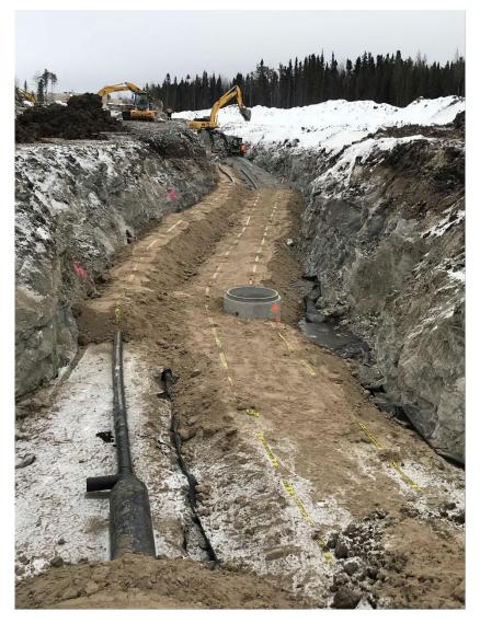
Over the next week pipping will continue to be installed from the onsite lift station towards the off-site tie in. The mainline pipe installation should be completed in approx. 10-14 days with the service lines, valves and hydrants being completed approximately 7 days after that. The onsite lift station will be completed in conjunction with the offsite metering chambers, lift station and truck fill building which should be commencing the first week of December.
