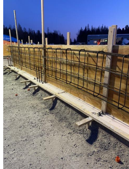
Rebar and Formwork for Concrete Grade Beam
