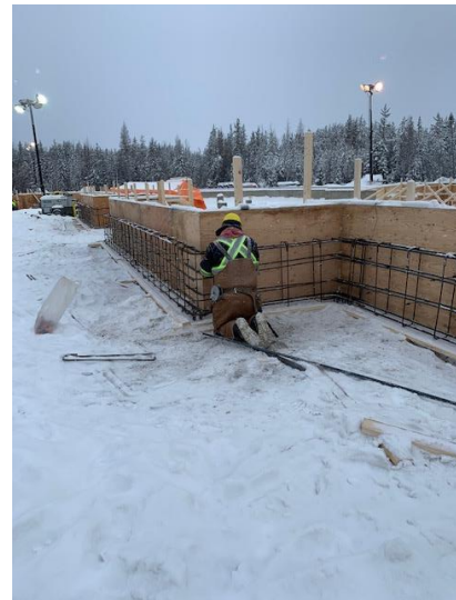
Installing Rebar for Grade Beam
