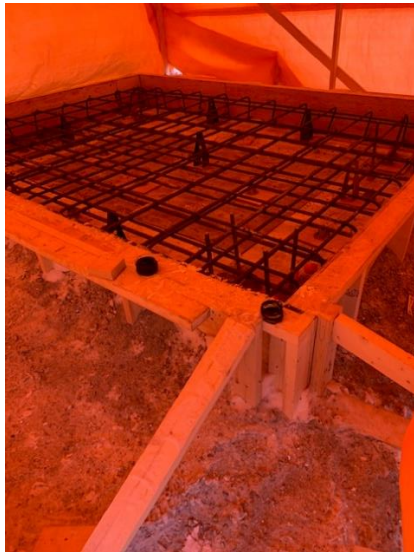
Rebar and Formwork for Elevator Pit Slab
