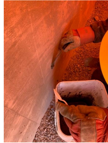
Grout tie holes in grade beam
