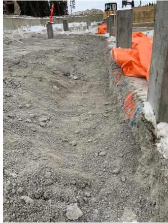
Trench for weeping tile in crawlspace
