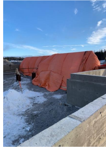
Hoarding and heating grade beam for pathing tie holes
