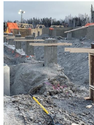
Support member for center beam formwork
