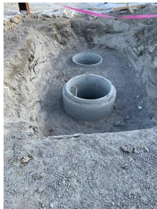
Sump Pit base installed
