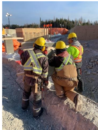
Construct support for center beam formwork
