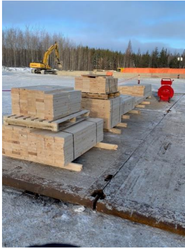
Pre-cut and stack framing materials
