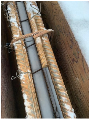
Rebar Install for center beam
