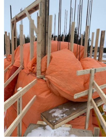
Hoarding and heating elevator shaft formwork
