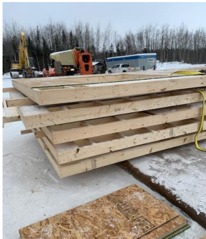
Prefab exterior wall sections
