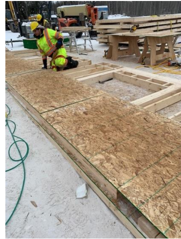
Construction of prefab exterior wall sections
