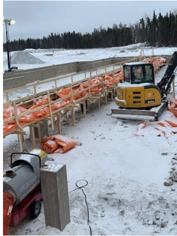
Heat and hoard formwork for center beam
