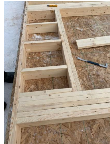
Construction of prefab exterior wall sections
