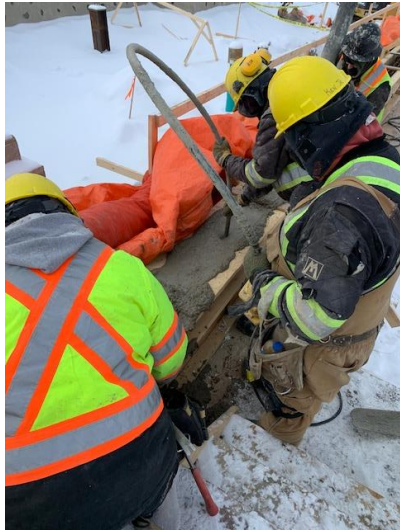
Vibrate concrete for center beam
