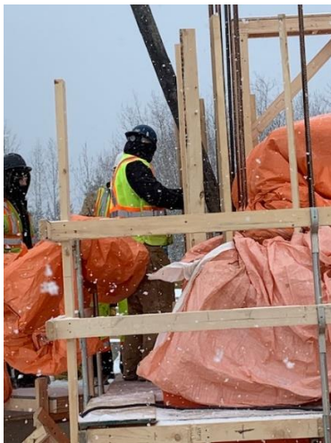
Pour concrete in elevator shaft formwork
