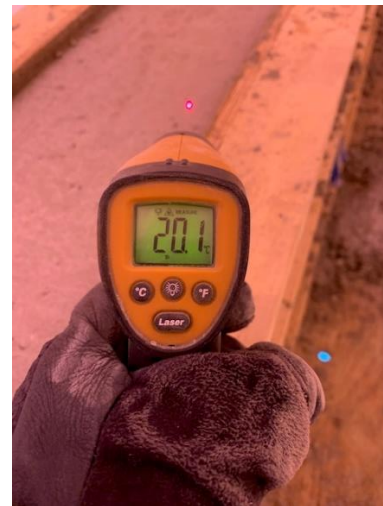
Verify concrete cure temperatures
