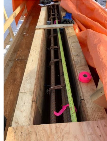
Verifying rebar spacing in center beam
