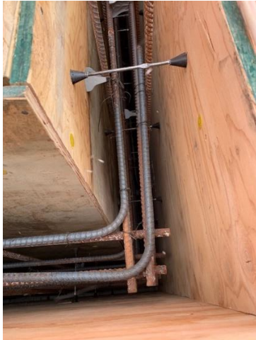
Verifying rebar spacing in elevator shaft
