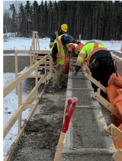
Verify top elevation of concrete center beam
