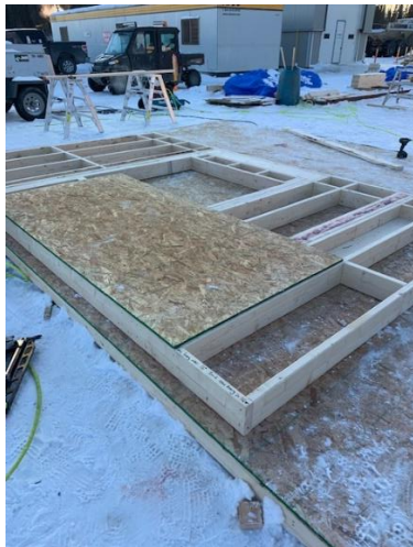
Prefab exterior wall section
