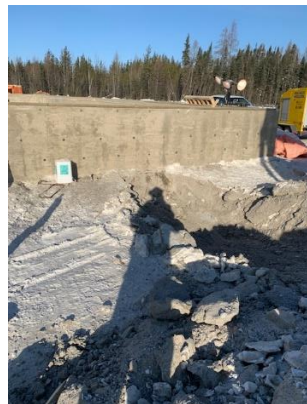
Trench for weeping tile
