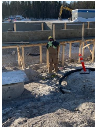
Remove formwork, walkway and supports from center beam
