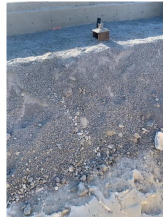
Backfill crawlspace
