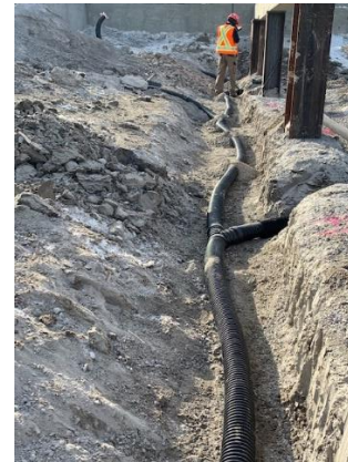
Weeping tile install in crawlspace
