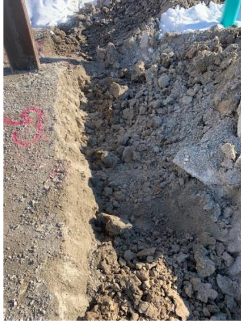
Trench for weeping tile
