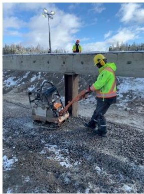
Compact backfill
