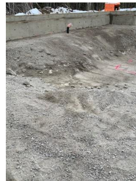
Backfill crawlspace
