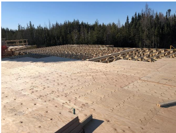
Second Floor Sheathing Install
