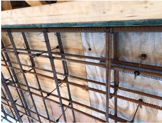
Elevator Shaft Rebar Install
