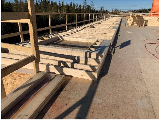
Second Floor Exterior Wall Framing
