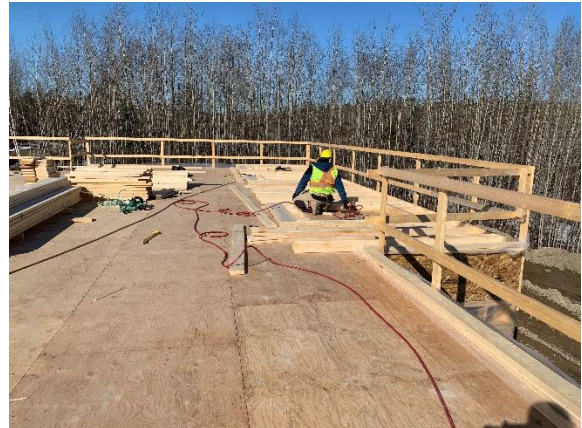
Second Floor Exterior Wall Framing
