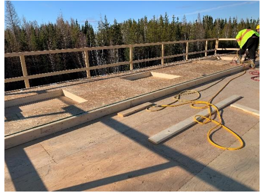
Second Floor Exterior Wall Sheathing
