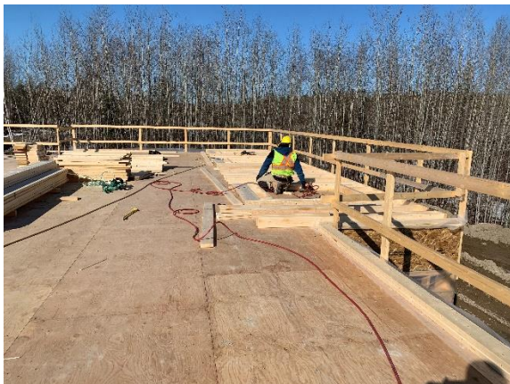
Second Floor Exterior Wall Construction
