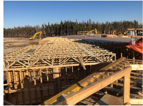
Second Floor Wood Truss Install
