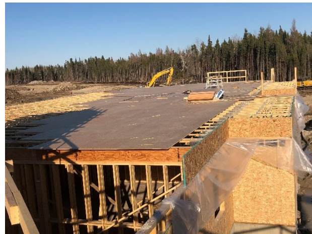
Rim Board and Poly Install
