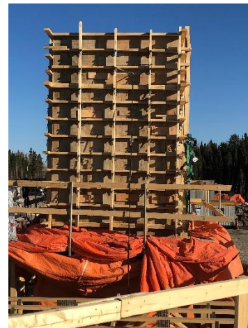
Elevator Shaft Formwork
