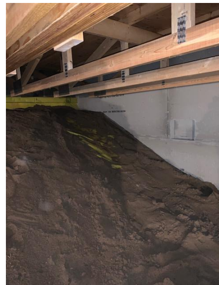
Crawlspace Fire Stop Wall
