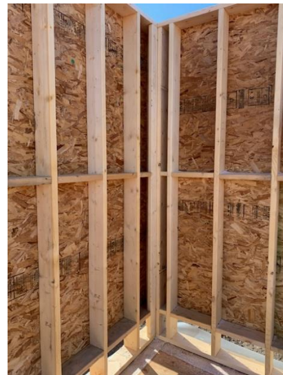
Second Floor Exterior Wall - Outside Corner
