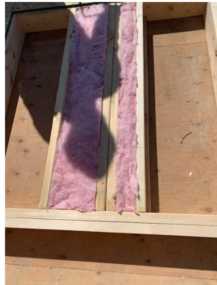
Second Floor Exterior Wall - Insulation
