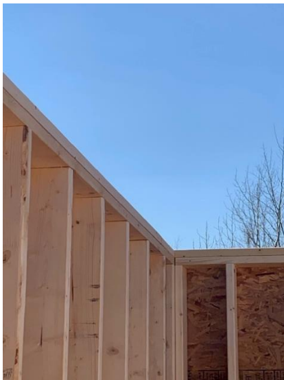
Second Floor Exterior Wall – Double Top Plate
