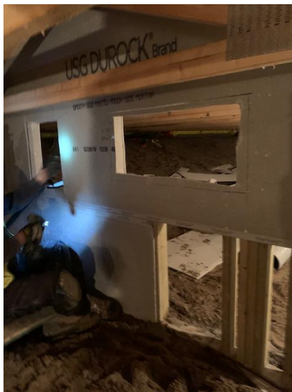
Crawlspace Fire Stop Wall - Ductwork openings
