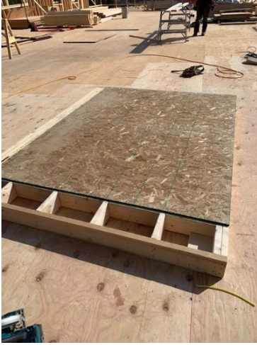
Second Floor Exterior Wall Sheathing
