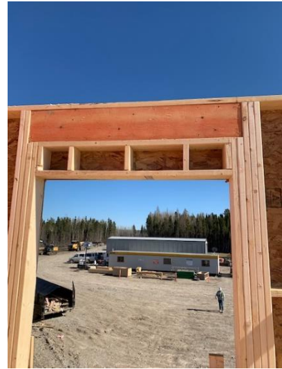
Second Floor Exterior Window - Lintel
