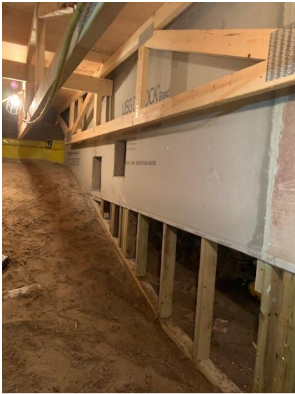
Crawlspace Fire Stop Wall - Cement Board Install
