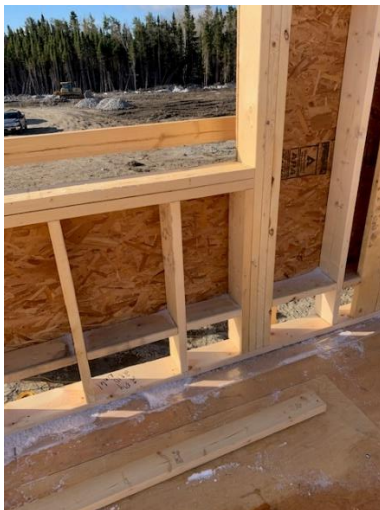
Second Floor Exterior Window - Sill - Jamb Detail
