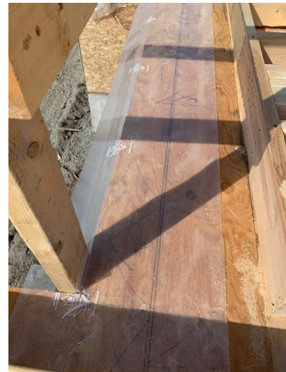
Second Floor Exterior Wall - Vapour Barrier
