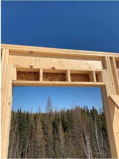
Second Floor Exterior Window - Header
