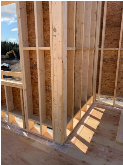
Second Floor Exterior Wall - Interior Corner
