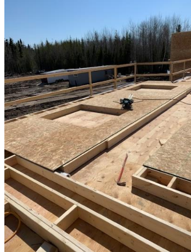
Second Floor Exterior Wall Sheathing
