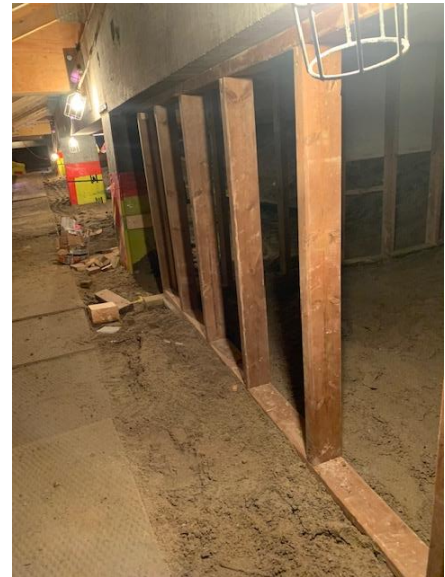
Crawlspace Fire Stop Wall - Framing
