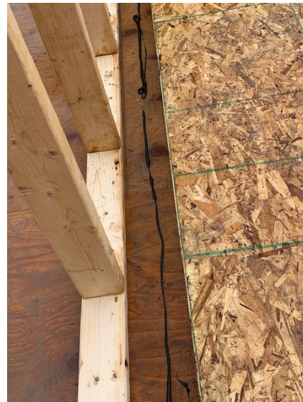
Acoustic Sealant Applied under Interior Demising Wall – West Side
