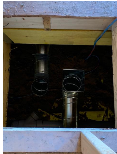
Duct Work Risers Leading to Main Floor West End
