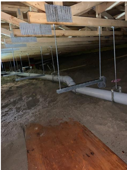
Main Sanitary Line Install with Hanger In Crawlspace – East Side
