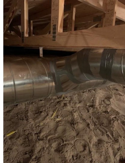
Duct Work Branch Line Installation in Crawlspace – West Side
