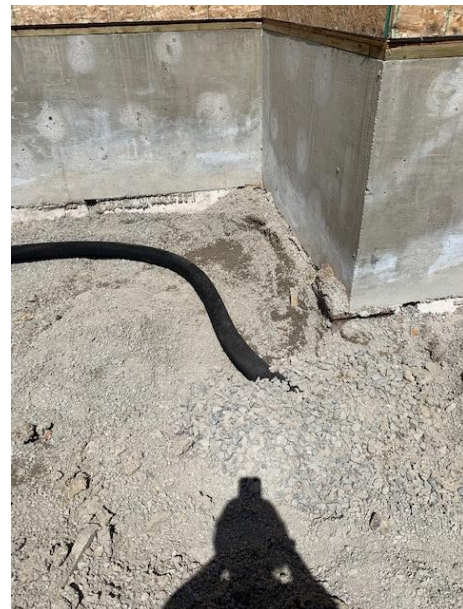
Exterior Weeping Tile Installation
