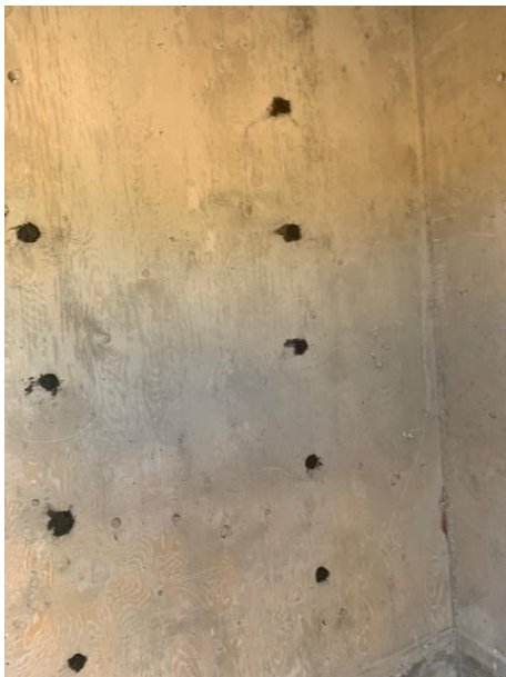
Grout Tie Holes – Interior Elevator Shaft Wall
