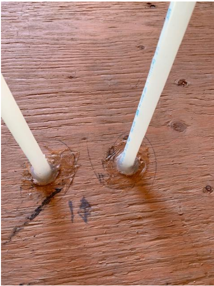
Seal Domestic Water Lines at Main Floor
