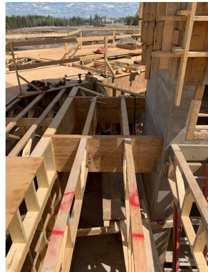
Second Floor Beam and Truss Install at Elevator - East Side
