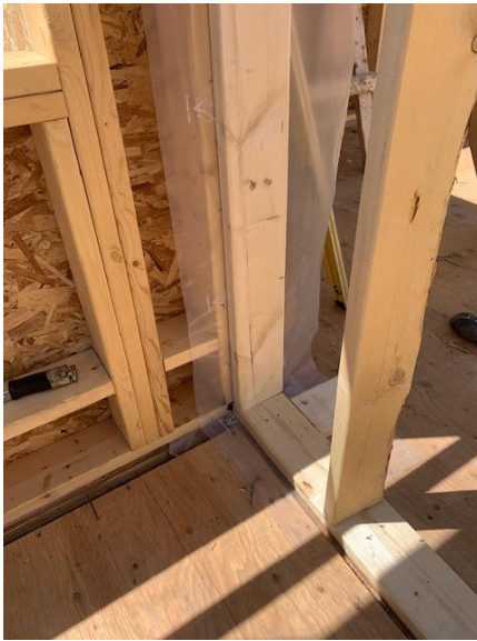
Vapour Barrier Install at Exterior Wall And Interior Corridor Wall – West End
