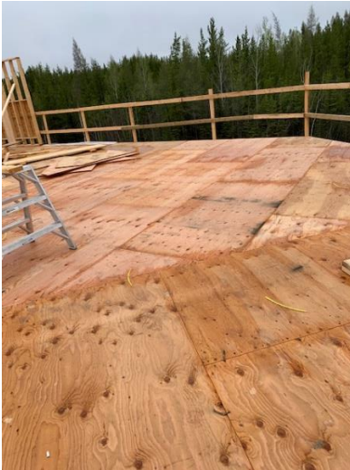
Second Floor Sheathing Install - North Side
