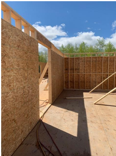
Corridor and Demising Wall Installation West Wing
