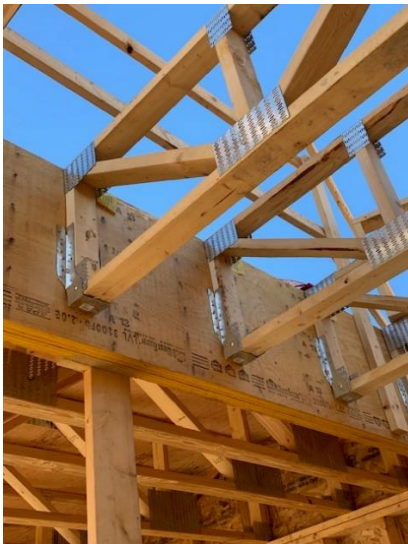
Second Floor Beam and Truss Install at Elevator – West Side
