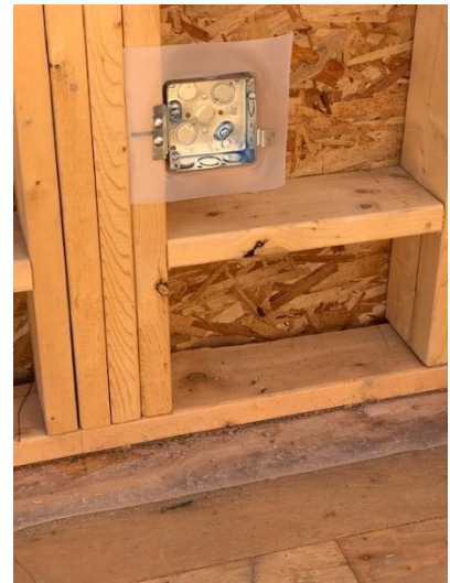
Electrical Box Install on Second Floor Suite Exterior Wall – West Wing
