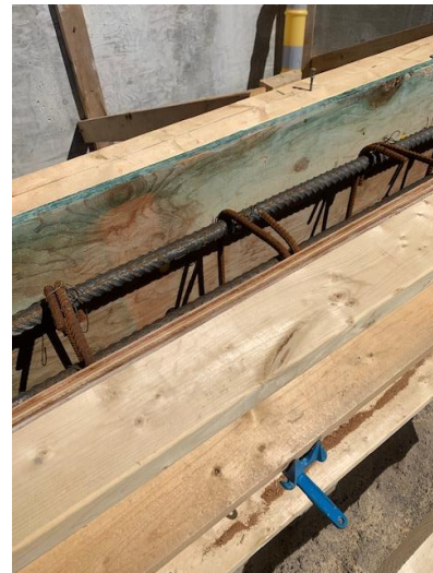
Formwork and Rebar Install for Main Entrance Beam
