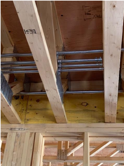
Conduit Install in Suite Ceiling on Main Floor West Wing
