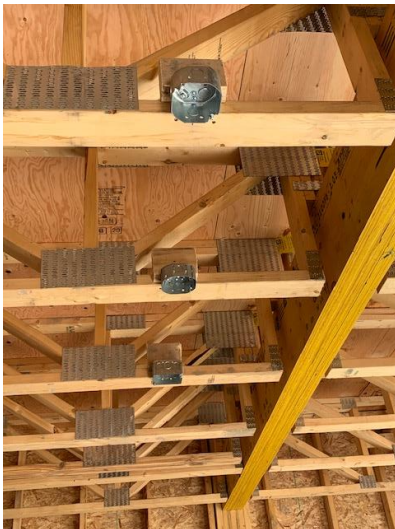
Electrical Boxes Mounted on Main Floor Suite Ceiling – West Wing
