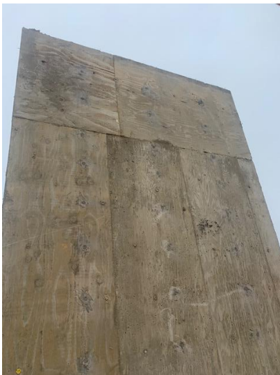
Grout and Smooth tie holes Exterior Elevator Shaft Wall – North Side
