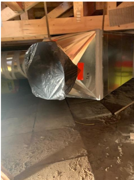
Duct Work Install in Crawlspace with Open Ends Protected – East Wing
