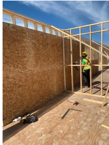
Second Floor Interior Corridor Wall Sheathing – East Wing
