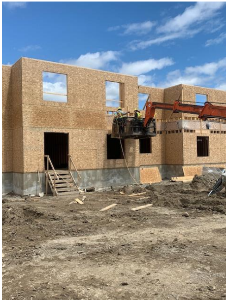
Exterior Sheathing Install Between Main And Second Floor – South East Side
