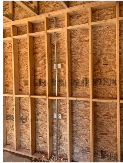
Conduit Install in Corridor Wall on Main Floor – West Wing
