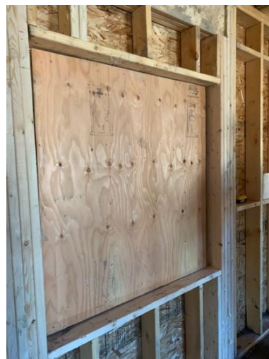
Electrical Panel Recess in Corridor Wall -Main Floor West Wing
