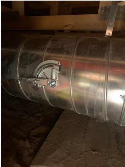
Duct Work with Damper Install in Crawlspace – East Wing
