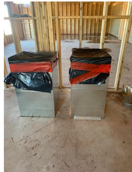
Duct Work Penetration Through Main Floor in Mechanical Room
