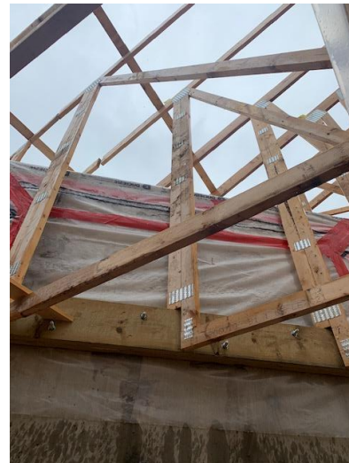
Roof Truss Install at Elevator Shaft
