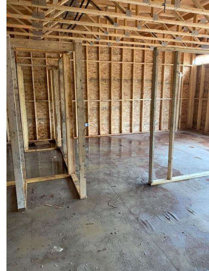
Temp Walls Install for Mock-ups
