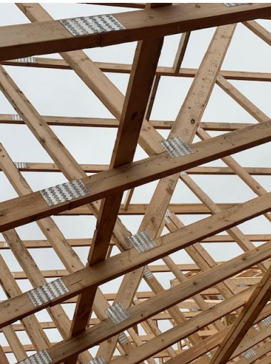
Roof Truss Bracing Install
