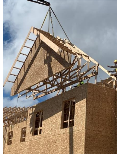
Raising Gable End Section
