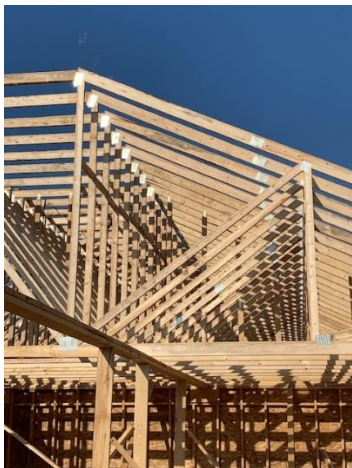
Roof Truss Install – West Wing
