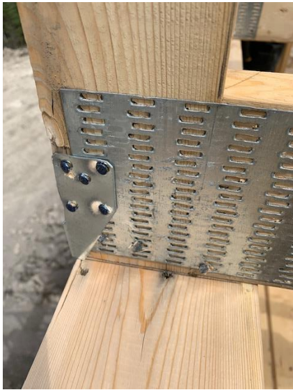
Roof Truss Tie Install
