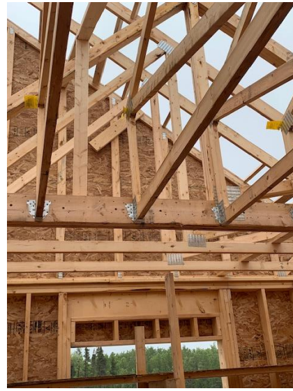
Roof Truss Hangers Install
