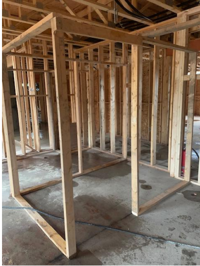
Temp Wall Install for Mock-ups
