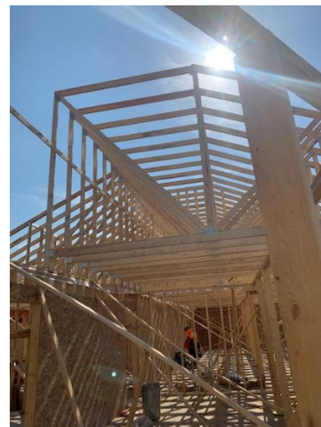
Roof Truss Install – East Wing
