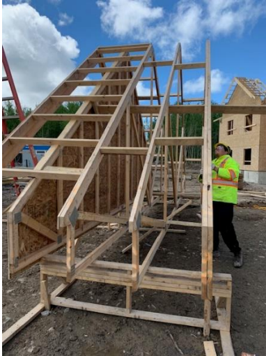
Framing Gable End Section
