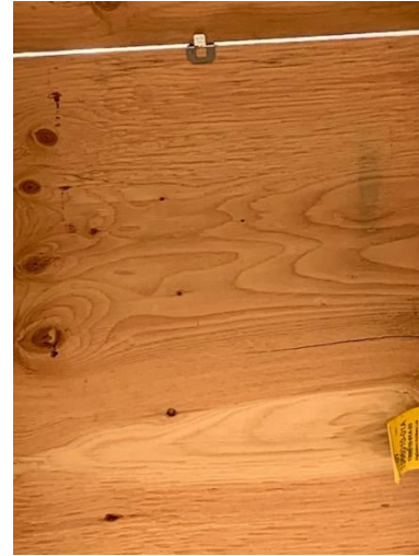
Roof Sheathing Clip Install – West Wing
