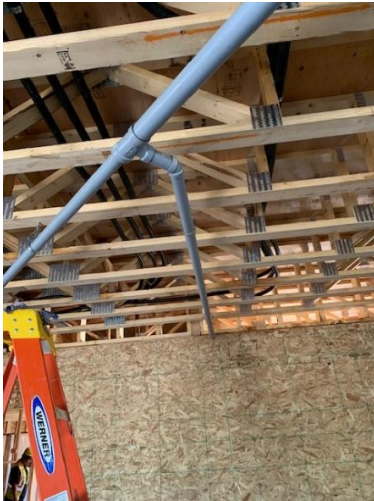
Plumbing Lines Install – Ceiling Laundry Room
