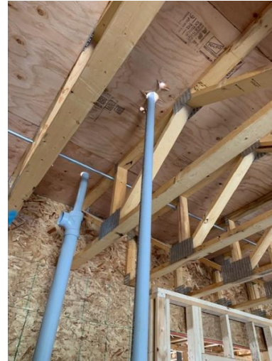
Plumbing Lines Install to Second Floor
