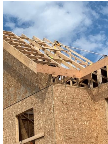
Gable End Truss Install – West Wing
