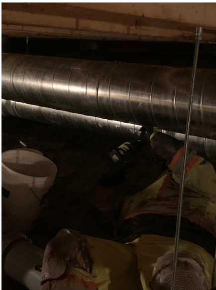
Duct Work Install in Crawlspace – East Wing
