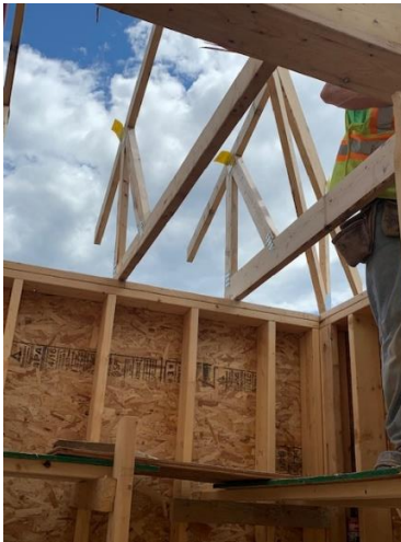
Roof Truss Install – East End
