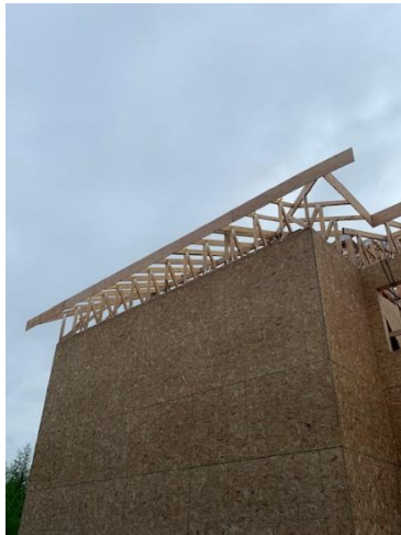
Fascia Board Install – West Wing
