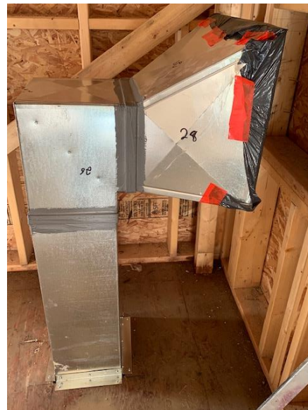
Duct Work Install at Stair No 2-West End
