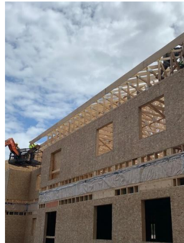
Fascia Board Install – North West Wing
