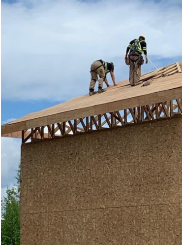
Roof Sheathing Install – West End
