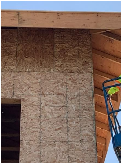
Exterior Sheathing Install – South East Wing
