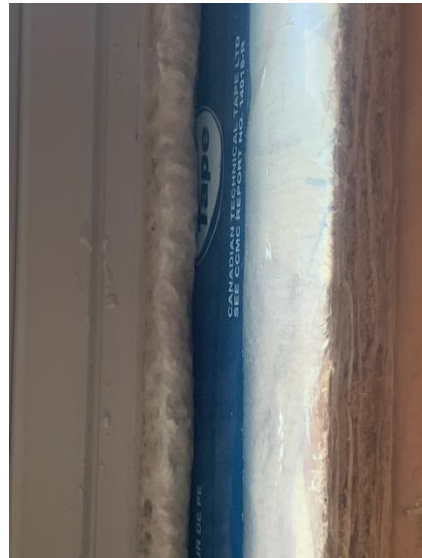
Spray Foam Insulation Applied for Window Mock-up – Top stair No. 3
