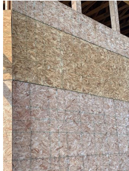
Exterior Sheathing Install – North West Wing
