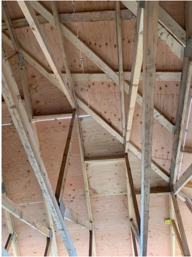
Roof Truss Bracing Install – East Wing
