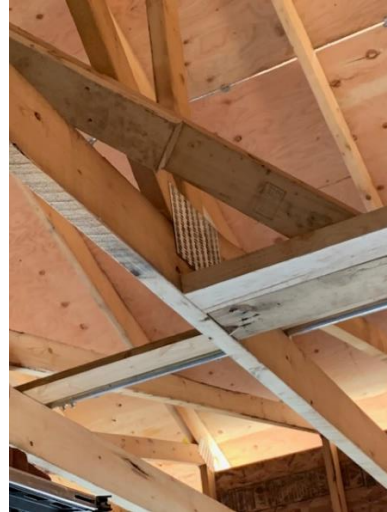
Roof Truss Bracing Install – West Wing
