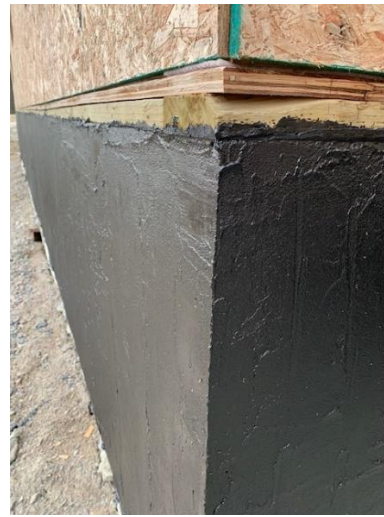
Foundation Coating Applied to Grade Beam
