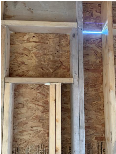
Framing for Duct Work Opening – Electrical Room
