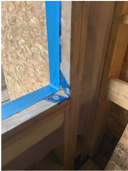
Blueskin and Vapour Barrier Install for Window Mock-up – Top Stair No. 3
