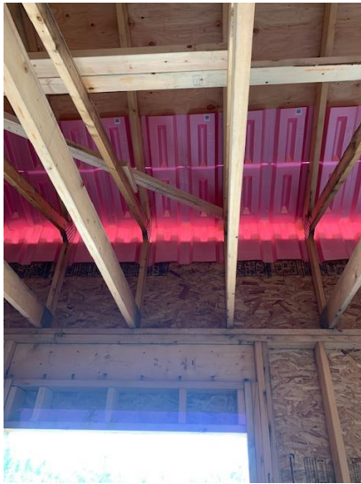
Attic Insulation Baffles Installed— North East Wing
