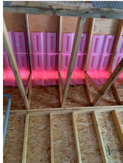
Attic Insulation Baffles Installed— South West Wing
