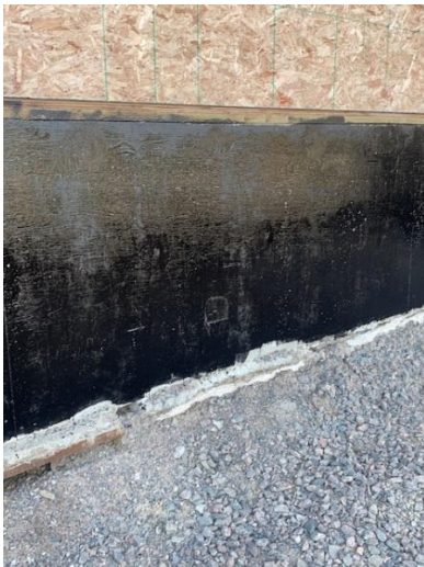
Primer Applied to Grade Beam
