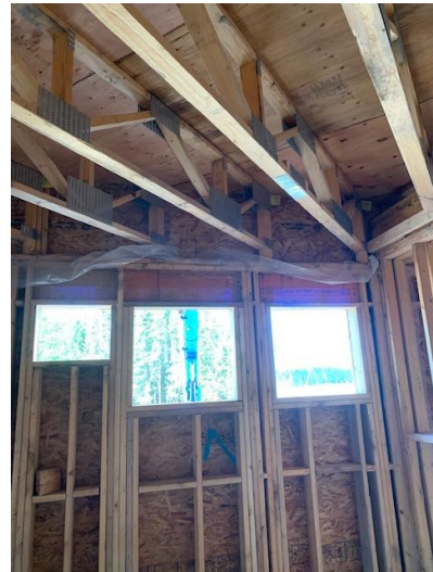
Framing for Duct Work Openings- Mechanical Room
