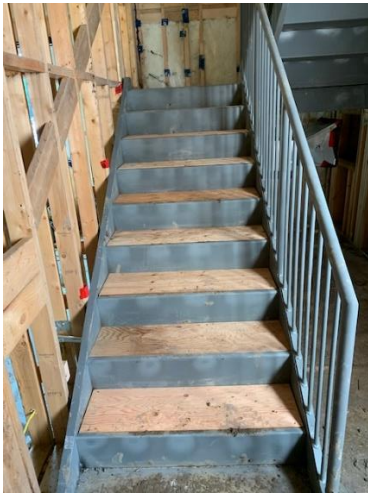
Temporary Steps Install on Stair No. 3
