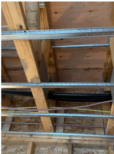
Resilient Channel Install on Main Floor Corridor Ceiling – West Wing
