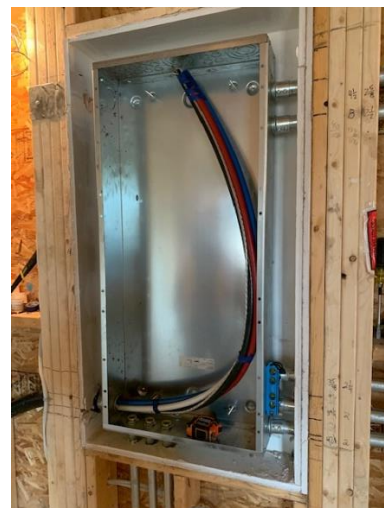
Electrical Panel Install in Corridor Recess on Main Floor – West Wing
