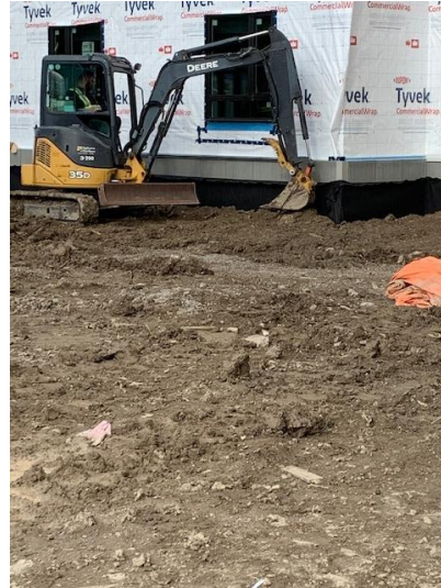
Backfill Around Foundation Wall – South West Wing
