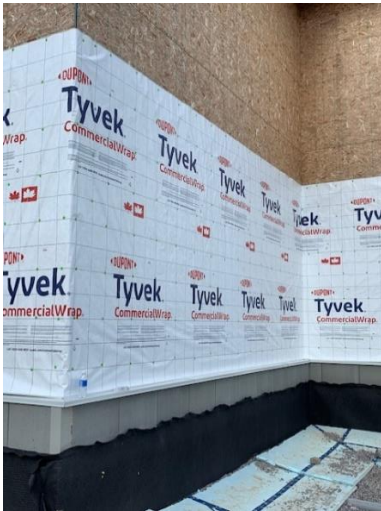
Commercial Wrap Installation – South East Wing
