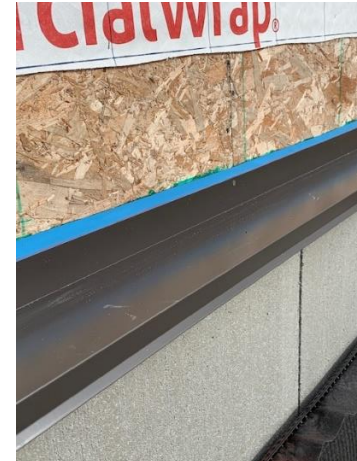
Flashing Installation over CFI Panels - South East Wing
