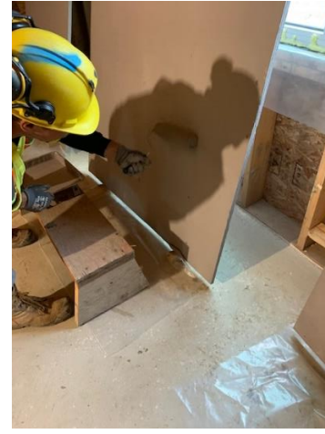
Paint Backer Boards for Electrical Panels
