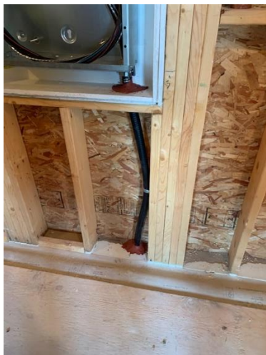
Fire Stopping Applied to Electrical Cables at recess Electrical Panel – Second Floor Corridor East Wing
