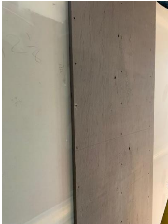
Install Backer Boards for Electrical Panels in Electrical Room
