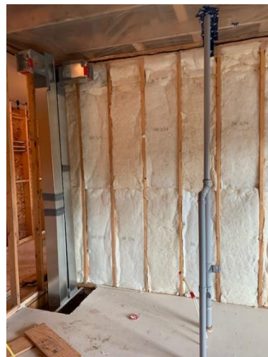
Batt Insulation Install on Second Floor Suite Wall (partial) – Suite 2Y:18
