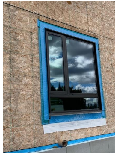
Blueskin Installation Around Window Frames – South East Wing
