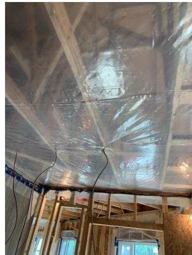
Vapour Barrier Install on Second Floor Suite Ceiling - Suite 2Y:18
