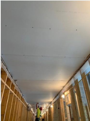
Gypsum Board Install on Second Floor Corridor Ceiling – West Wing
