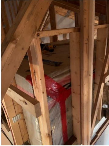
Wood Stud Wall Framed Around Elevator Shaft in Attic Space
