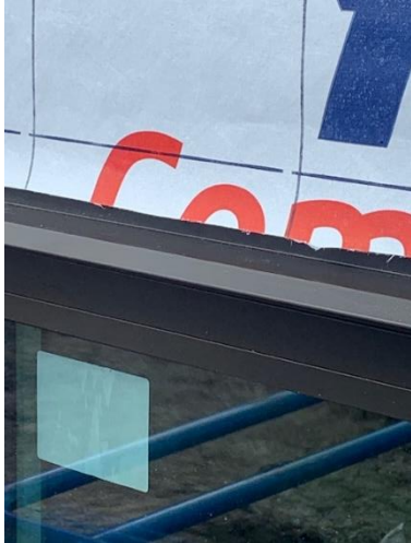
Above Window Flashing Install – South West Wing
