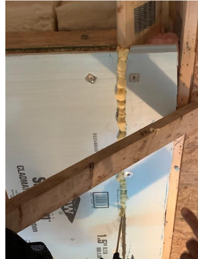
Batt and Rigid Insulation Installation on Elevator Roof and Shaft Walls
