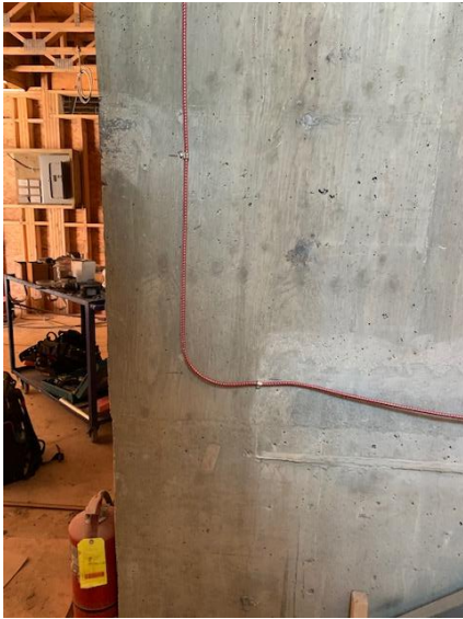
Electrical Wiring Install on Elevator Shaft Wall
