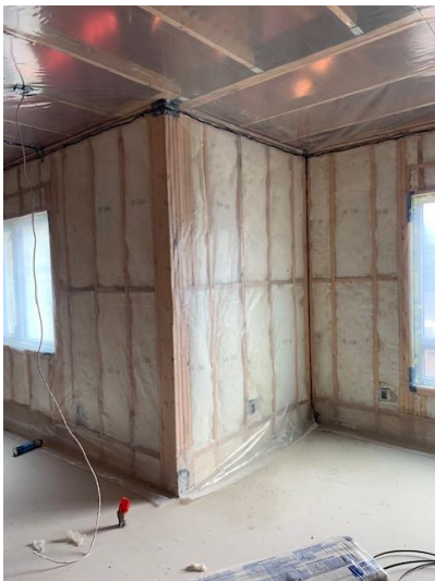
Batt Insulation and Vapour Barrier Install On Second Floor Exterior Walls – South West Wing
