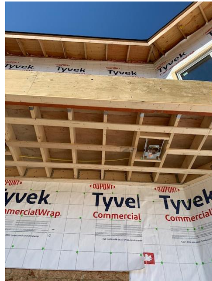
Electrical Lighting Box and Wiring Install In Ceiling of Front Canopy
