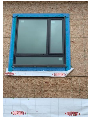
Blueskin Install Around Window Frame - North West Wing
