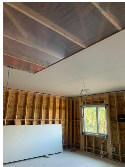
Gypsum Board Install on Second Floor Suite Ceilings – North West Wing
