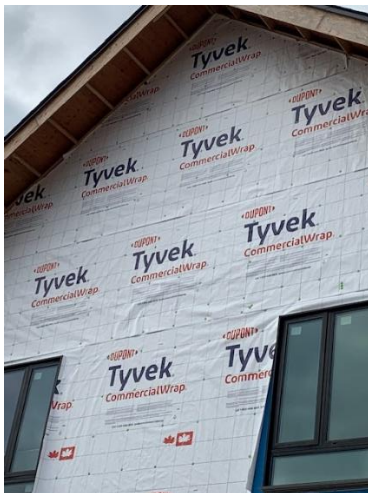
Commercial Wrap Install on Gable End – South East Wing
