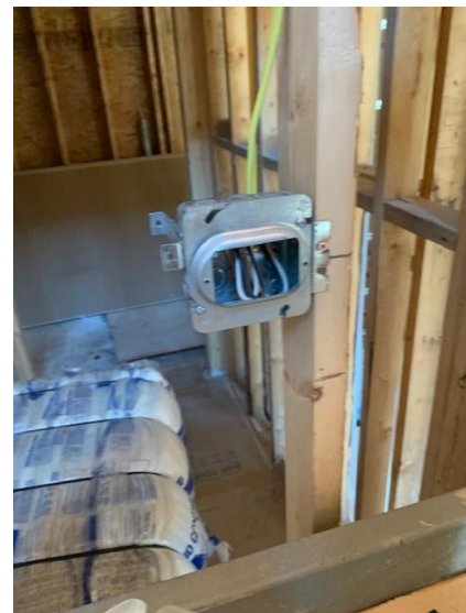
Electrical Box and Wiring Install at Stair No. 1
