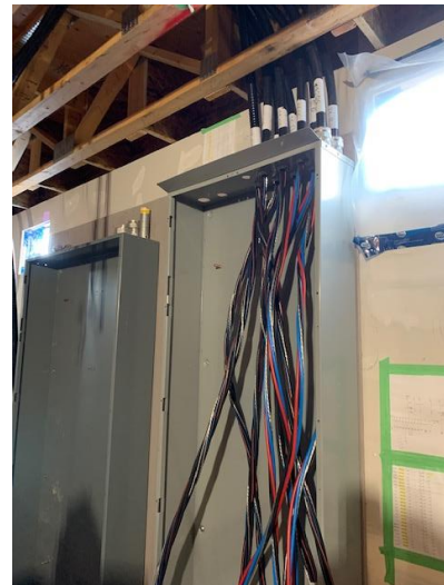
Electrical Wiring Install at Distribution Panel in Electrical Room
