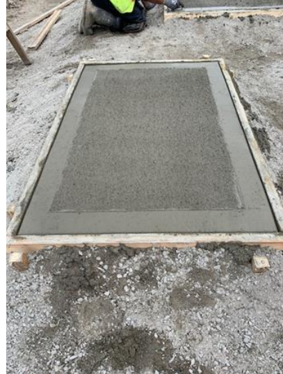
Mechanical Concrete Pads
