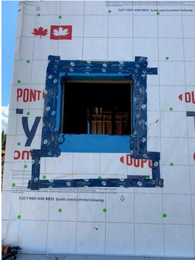
Blueskin Applied Around Exterior Openings – Stairwell No. 2
