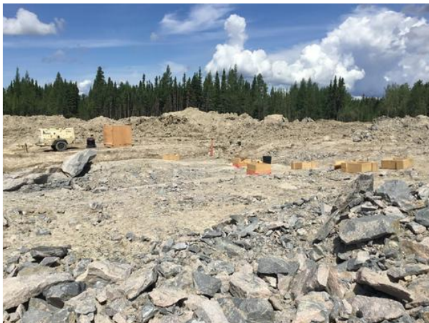
Footing formwork
