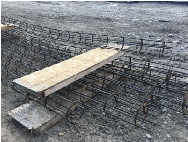
Completed rebar cages Hooman Kazempour Jul 22, 2020 1:57 PM
