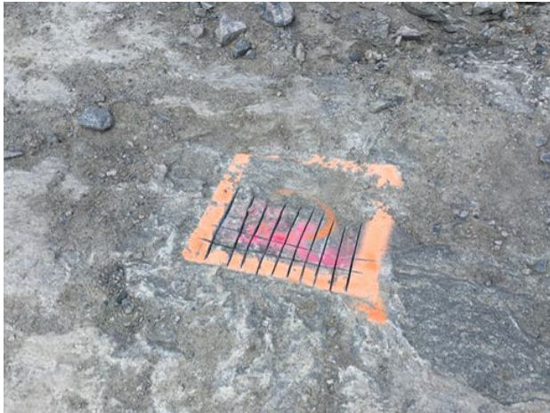
Footing location to be chipped
