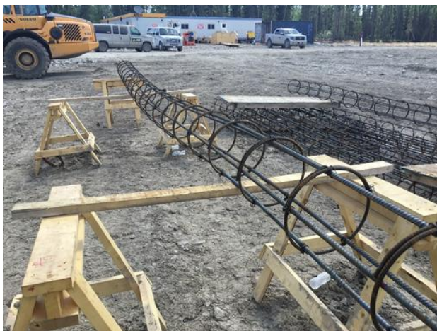
Rebar cages being tied Hooman Kazempour Jul 22, 2020 1:57 PM
