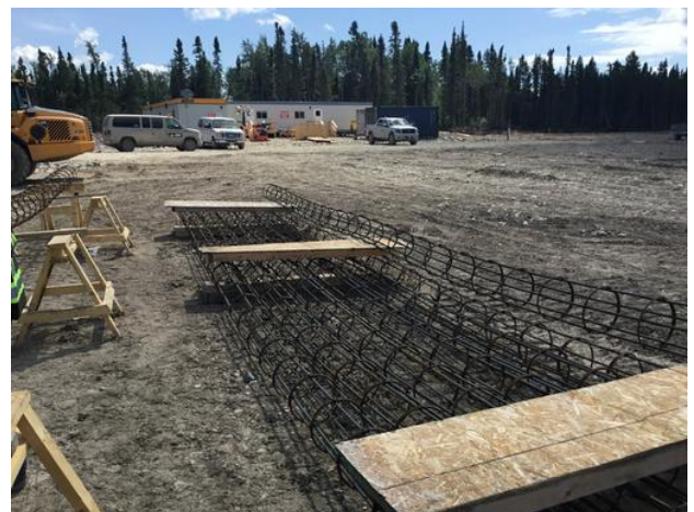
Completed rebar cages Hooman Kazempour Jul 22, 2020 1:57 PM
