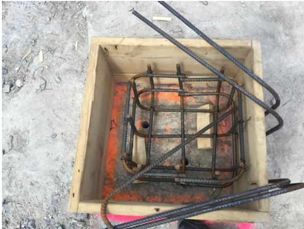
Rebar being placed in footing form work
