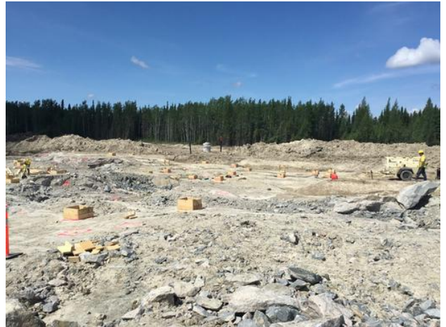
Footing formwork at various locations
