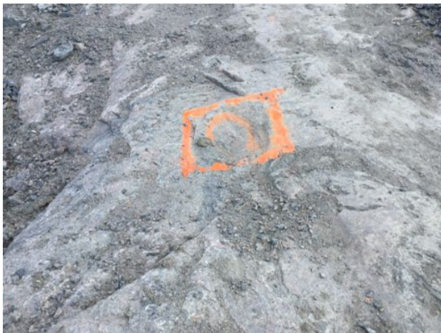
Footing location marked out
