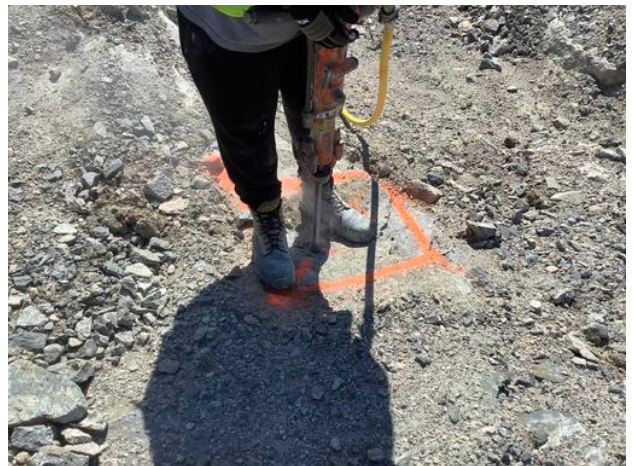
Drilling for pad locations
