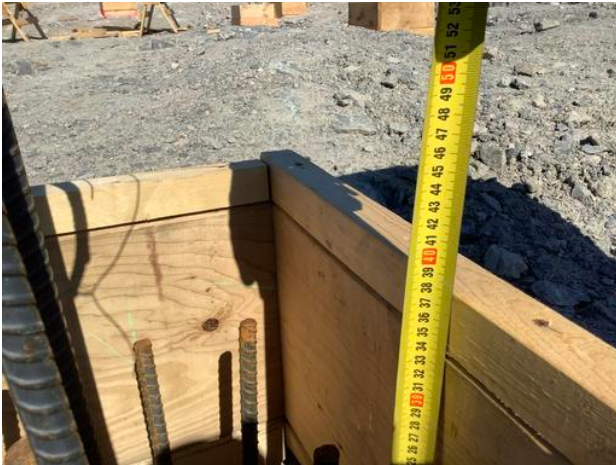
Footing formwork
