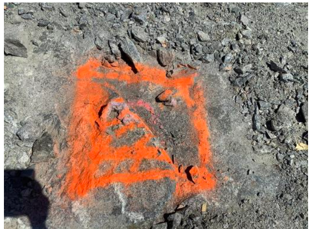
Footing location marked out
