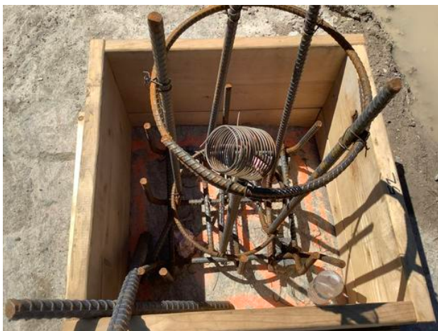
Rebar being placed in footing form work Wayne Dee Jul 30, 2020 2:11 PM
