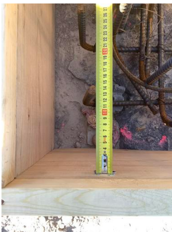
Footing formwork dimensions
