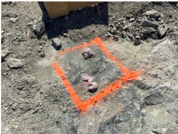
Footing location marked out
