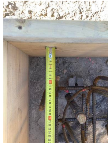
Footing formwork dimensions
