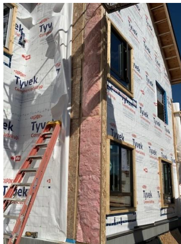
Batt Insulation Installation in Wing Walls – South West Wing
