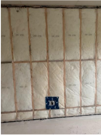
Batt Insulation and Vapour Barrier Install on Second Floor Exterior Walls - East Wing
