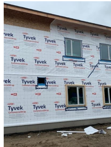
Commercial Wrap Install - North East Wing
