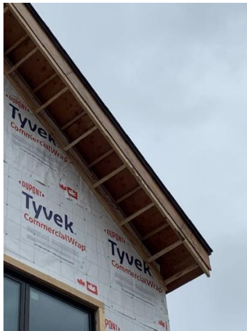
Gable End Soffit Framing – South East Wing
