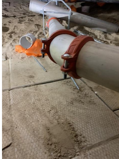
Main Water Service Line Install in Crawlspace
