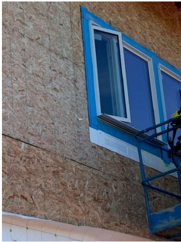
Blueskin Applied Around Window Frames – North East Wing
