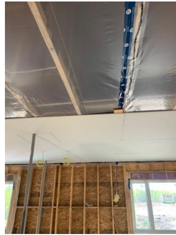
Gypsum Board Installation on Second Floor Suite Ceiling – Suite 2Y:11
