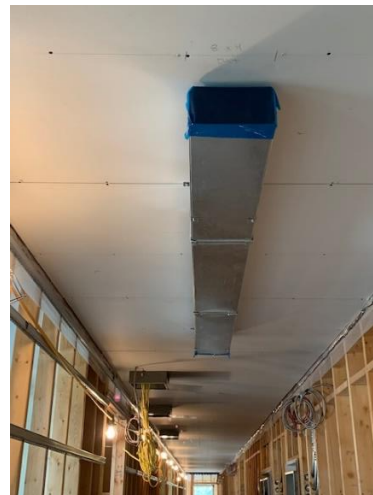
Duct Work Install on Second Floor Corridor Ceiling – West Wing
