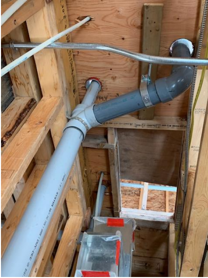
Plumbing Sanitary Lines Install to Second Floor – East Wing
