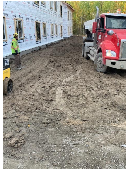
Backfill Around Foundation Wall – North West Wing
