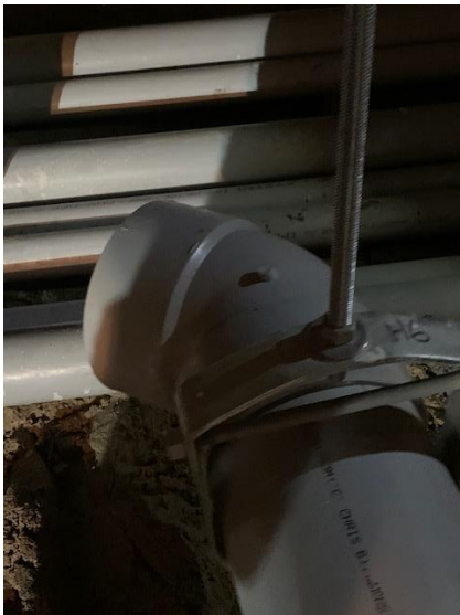
Main Sanitary Service Line Install in Crawlspace
