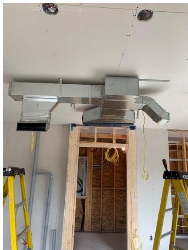
Duct Work Install on Second Floor Suite Ceiling – Suite 2Y:17
