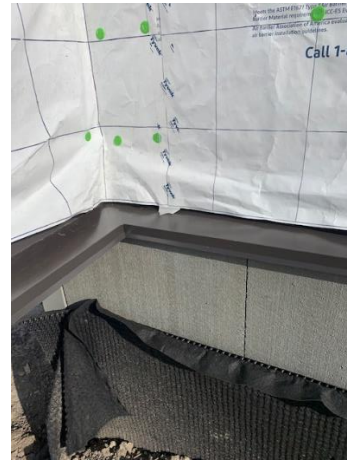
Flashing Install Above CFI Panels – South East Wing
