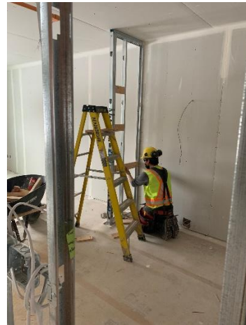
Wood Blocking Installation in Steel Stud on Second Floor – West Wing
