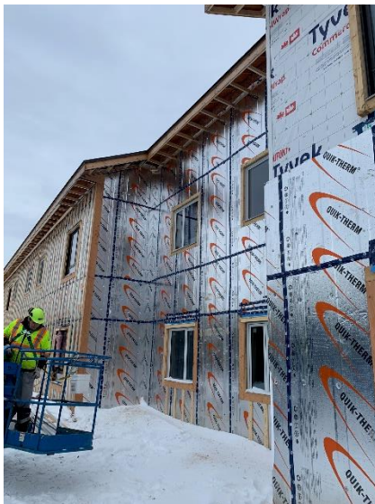
Exterior Rigid Insulation Install - North West Wing
