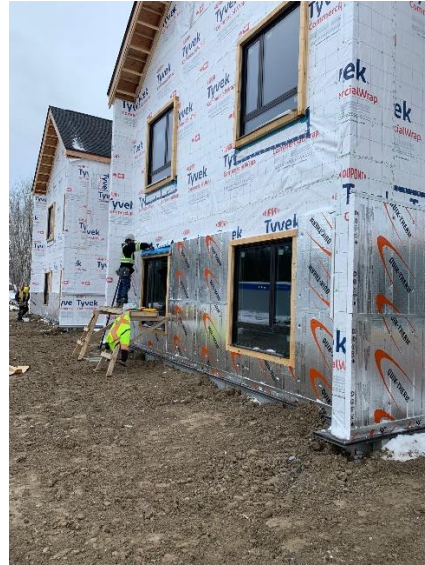
Exterior Rigid Insulation Install – South West Wing
