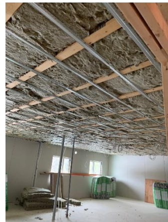
Resilient Channel Install on Main Floor Suite Ceiling – West Wing
