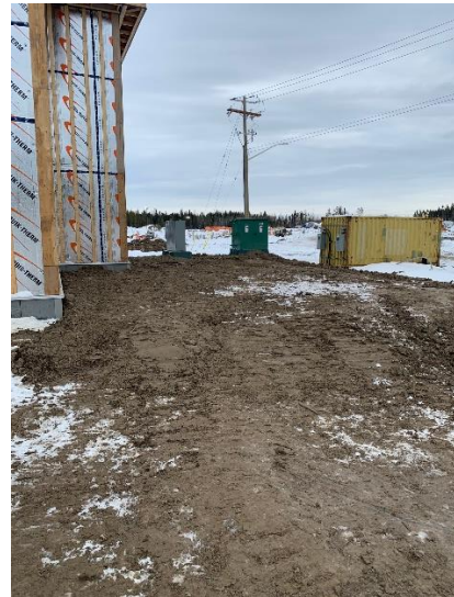
Backfill Around Foundation Wall – East End
