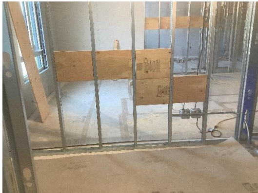
Wood Blocking Installatin in Steel Stud Wall On Second Floor – East Wing
