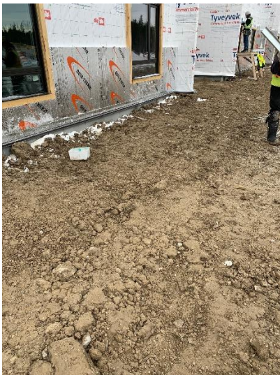
Backfill Around Foundation Wall - South West Wing
