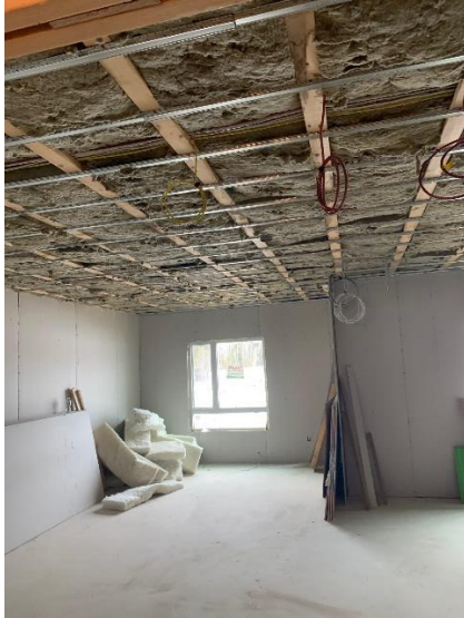
Rockwool Insulation Install on Main Floor Ceiling – East Wing
