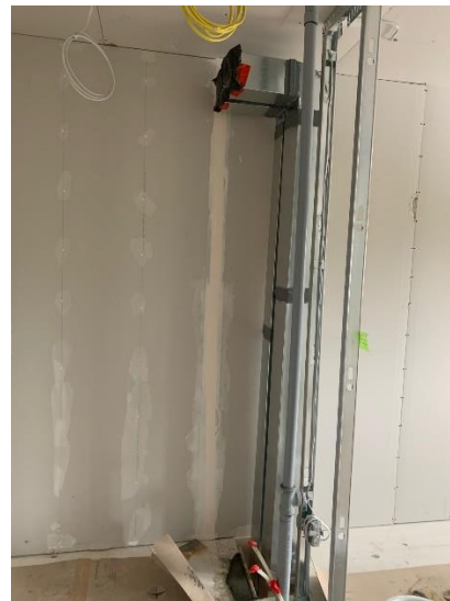
Drywall Tape and Mud Applied to Gypsum Board on Second Floor – West Wing
