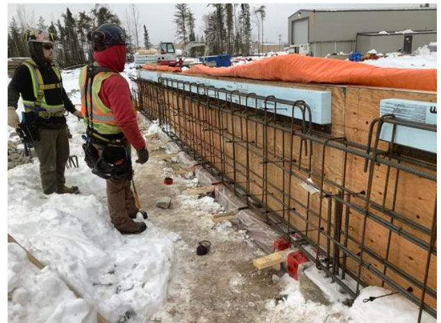
rebar install in grade beam formwork
