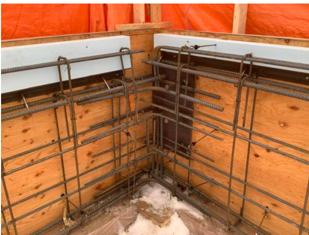
grade beam corner with steel embed
