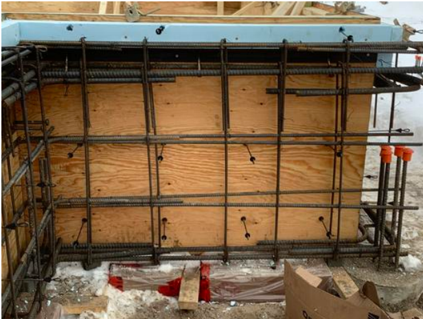
Grade beam formwork area A1 with steel angle
