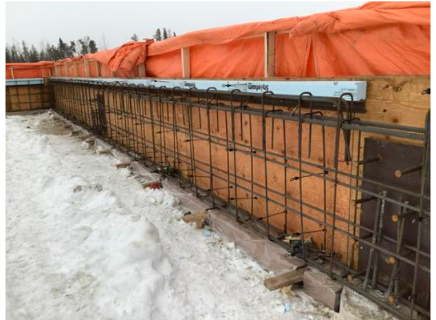
Grade beam formwork with rebar installed
