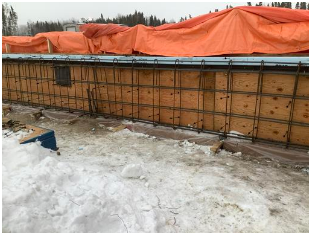
temp hoarding and grade beam formwork Wayne Dee Nov 3, 2020 11:43 AM
