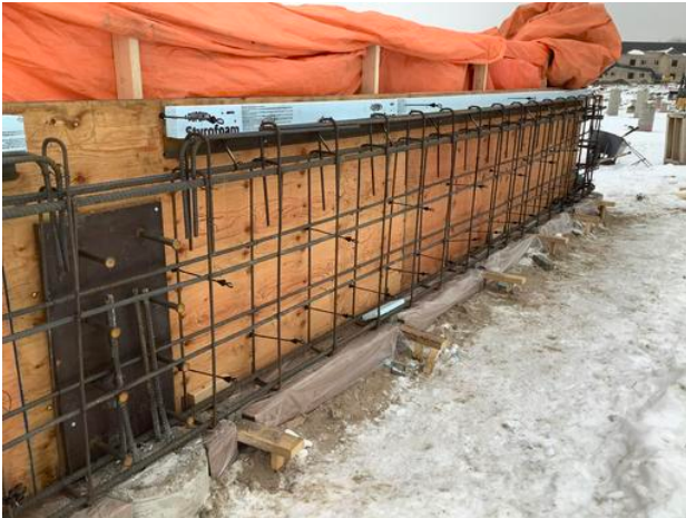
grade beam corner with steel embed
