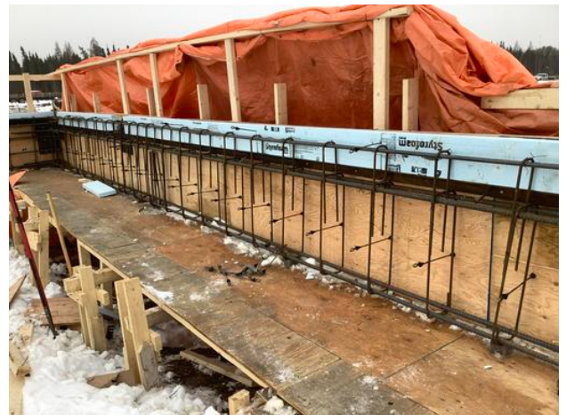
Grade beam formwork w/ hoarding being constructed
