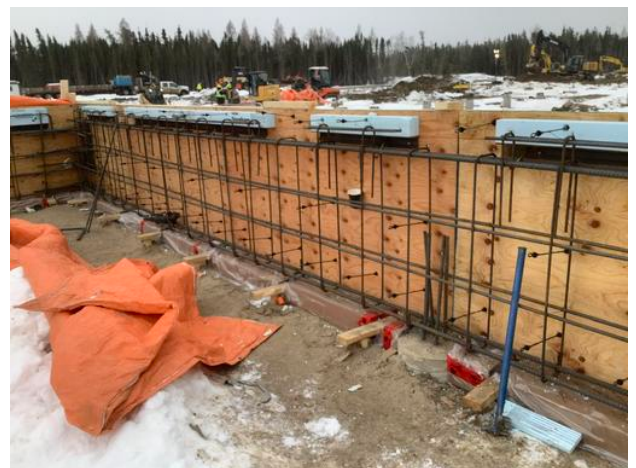
side view of grade beam formwork install Wayne Dee Nov 3, 2020 11:47 AM
