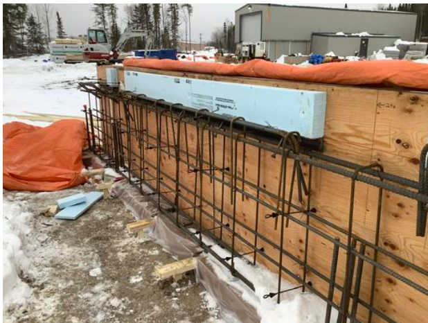
Rebar being placed in footing form work
