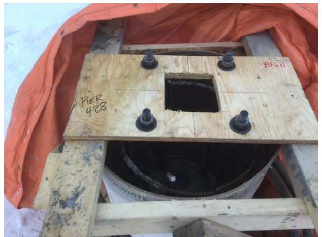
anchor bolts embed in pier formwork
