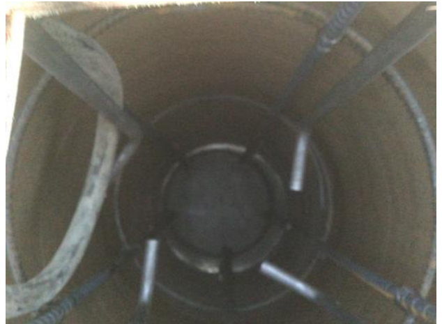
concrete pier rebar
