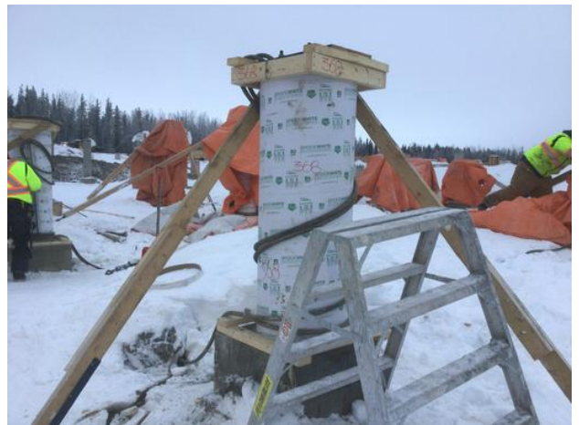
concrete pier formwork framing
