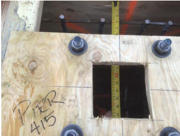
anchor bolts embed in grade beam formwork
