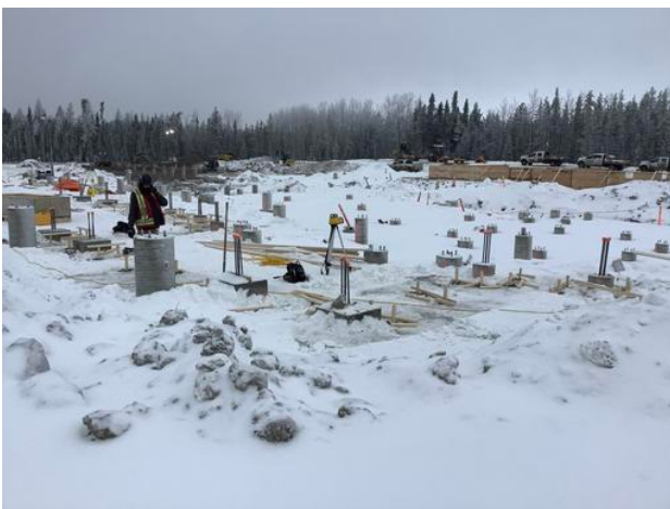
Preparation for pier forming
