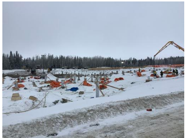
Concrete pump line pouring pads and piers
