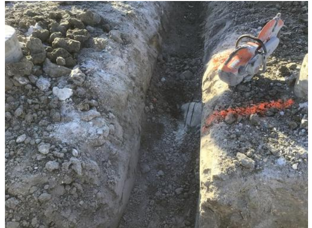
removing rock with quick saw in a trench run
