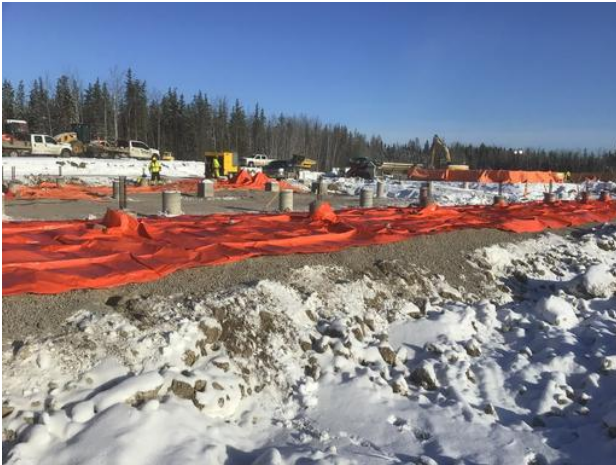
crawlspace poly install
