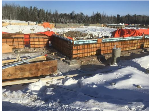
Grade beam formwork with rebar
