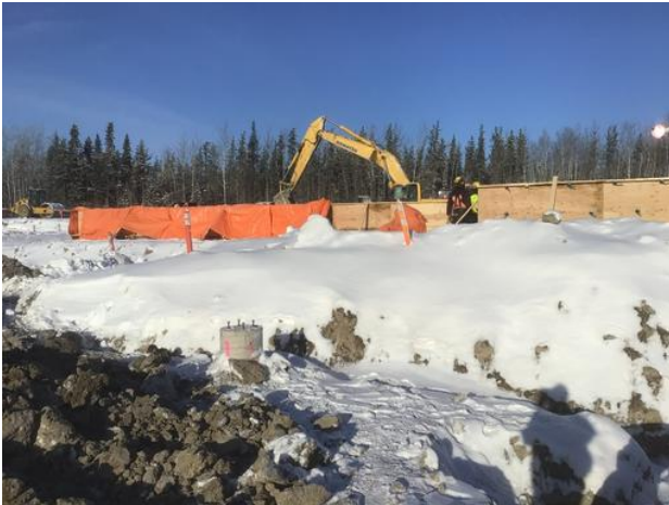
backfill operations past grade beam forming
