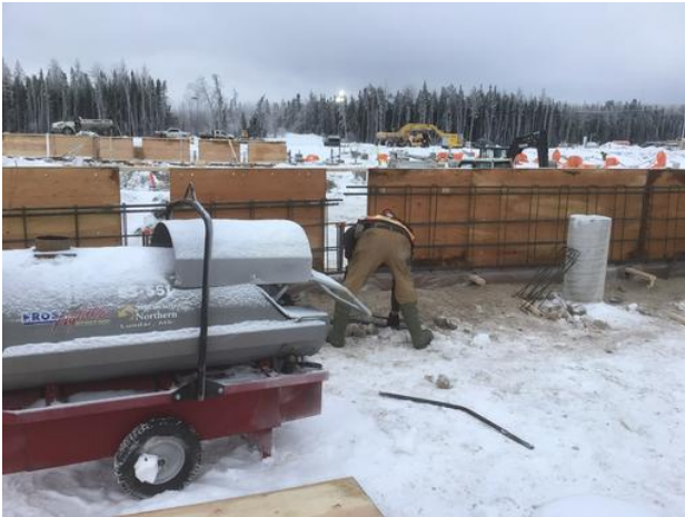
grade beam rebar install
