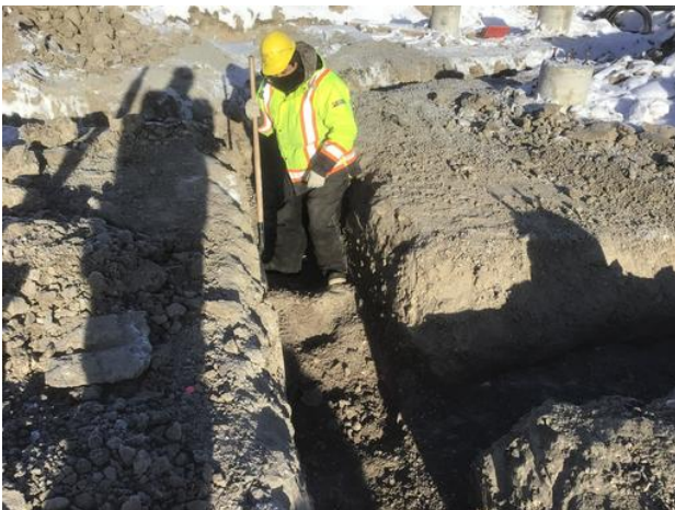
detailed hand excavation in trenches
