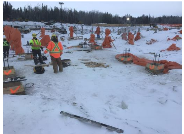
pad location rebar install
