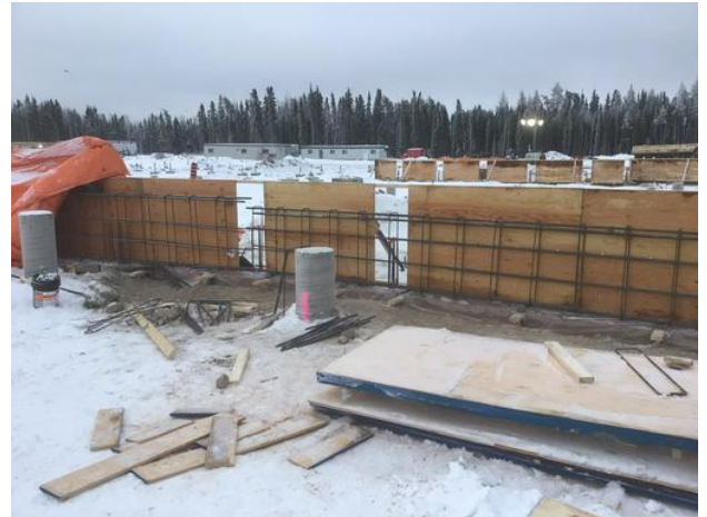
Grade beam formwork with rebar
