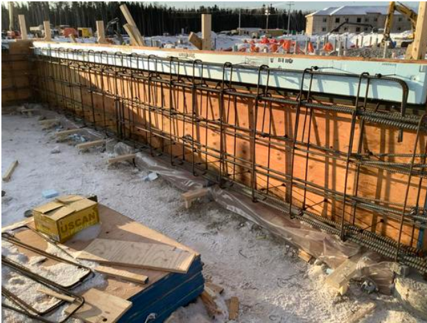
Grade beam formwork with rebar
