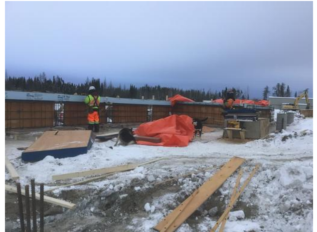
Grade beam formwork with rebar Wayne Dee Nov 22, 2020 3:23 PM
