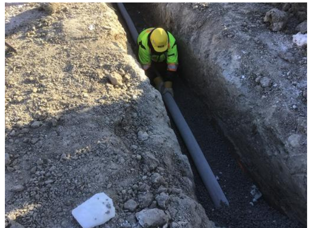
placing piping in trench
