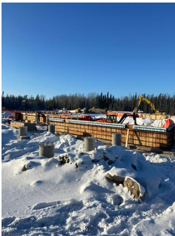
Grade beam formwork with rebar
