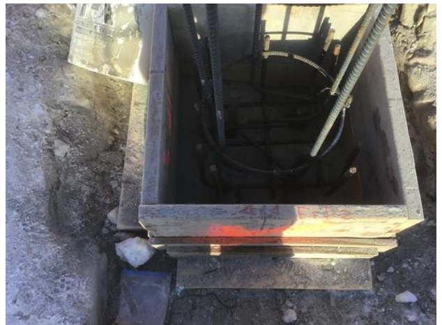
pier and pad rebar
