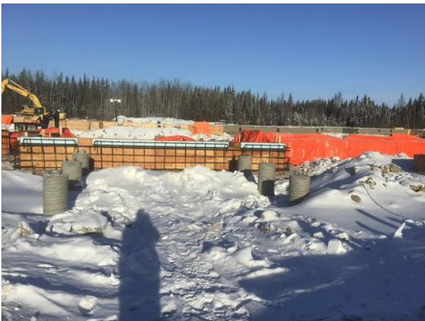
grade beam heating and hoarding
