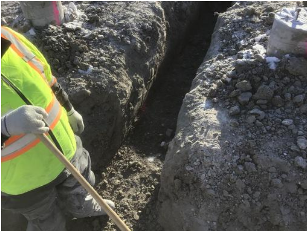
hand trenching for mechanical
