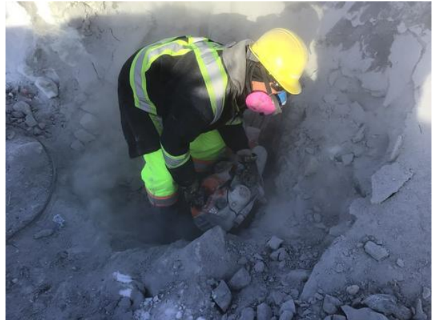
removing rock via quick saw
