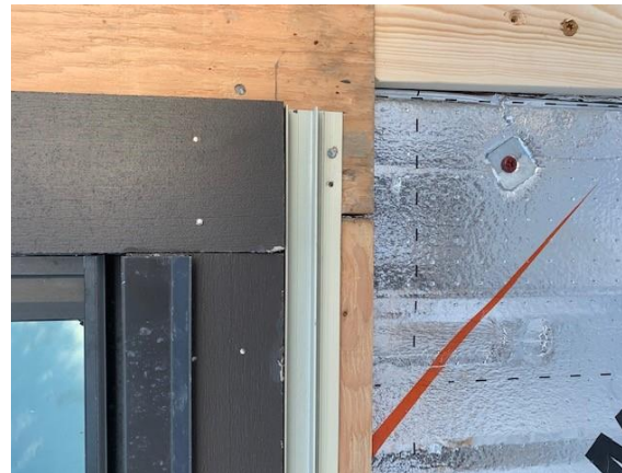
Fiber Cement Panel Trim Install - South West Wing
