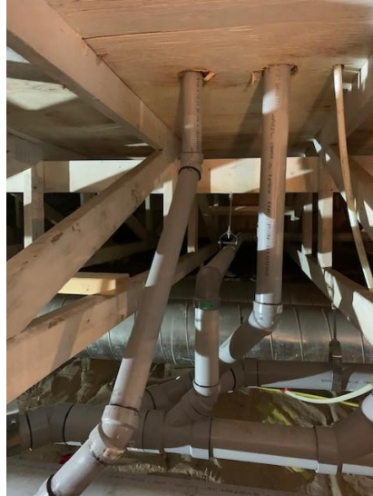
Sanitary Lines Install in Crawlspace - West Wing
