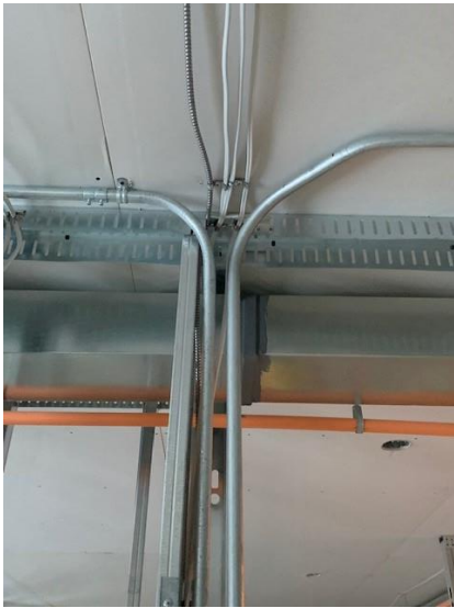
Electrical Conduit Install in Second Floor Suite – West Wing
