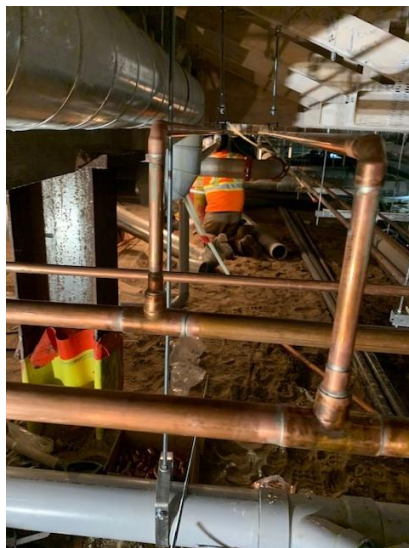
Domestic Water Line Install in Crawlspace – East Wing
