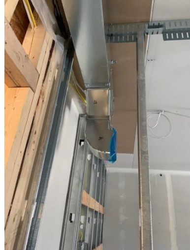
Ductwork Install on Second Floor – East Wing
