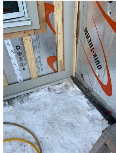
Lap Siding Trim Install - South West Wing
