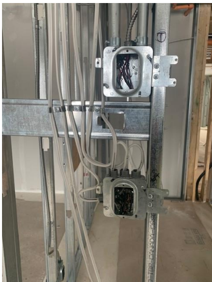
Electrical Box and Wiring Install in Second Floor Suite – East Wing
