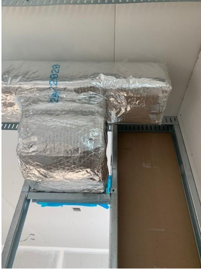
Ductwork Insulation Install on Second Floor – West Wing
