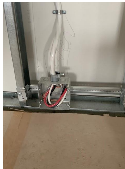
Electrical Box and Wiring Install in Second Floor Suite – West Wing
