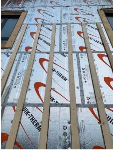
Exterior Strapping Install - South West Wing
