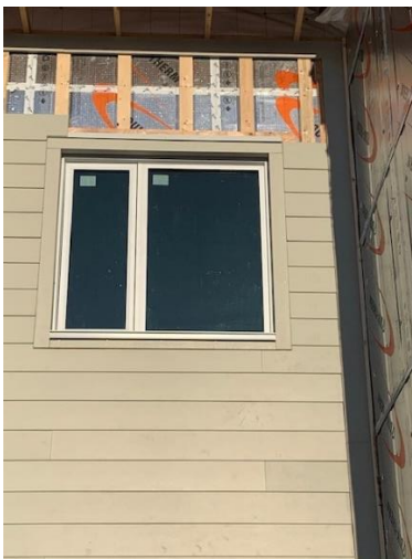
Lap Siding Install – South West Wing
