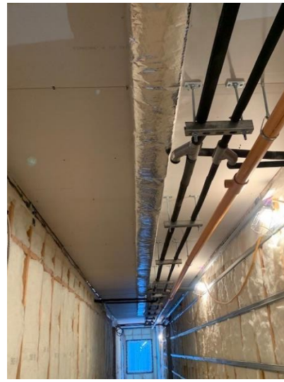
Ductwork Insulation Install on Second Floor Corridor – East Wing
