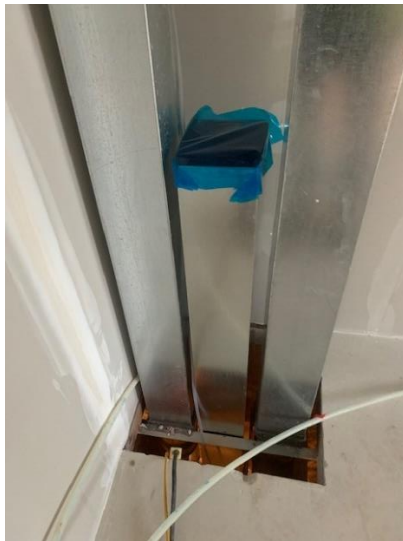
Ductwork Shaft Install from Crawlspace - East Wing
