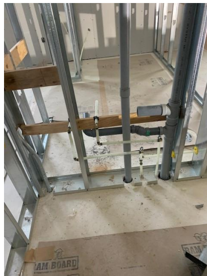
Domestic Water Line Install on Second Floor – West Wing
