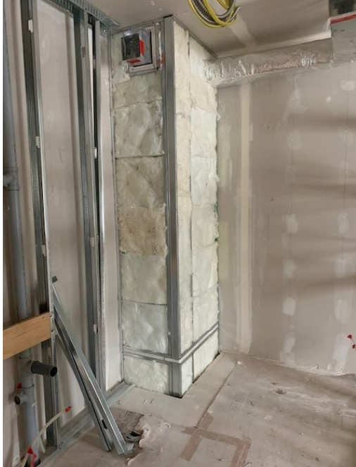
Mechanical Shaft Insulation Install
