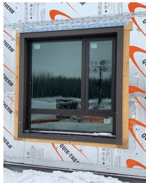
Fiber Cement Trim Installation
