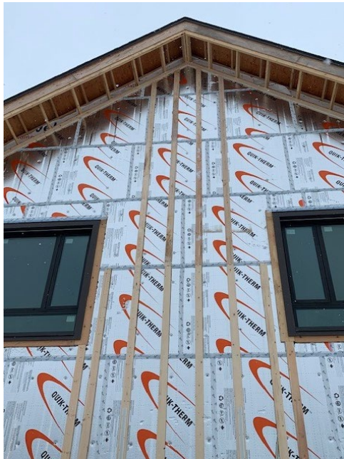
Exterior Strapping Installation
