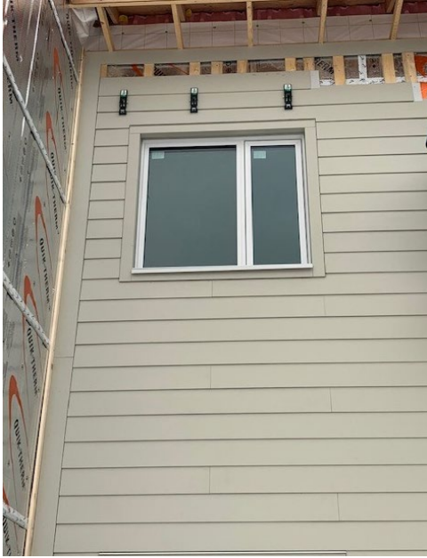
Fiber Cement Siding Install
