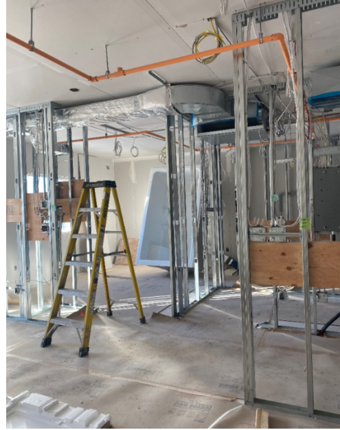
Steel Stud Framing Second Floor
