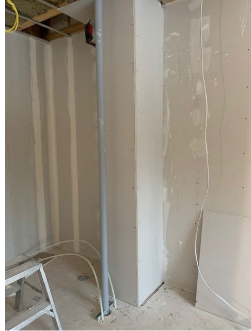
Mechanical Shaft Gypsum Board Install
