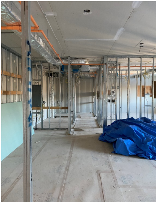
Steel Stud Framing Second Floor
