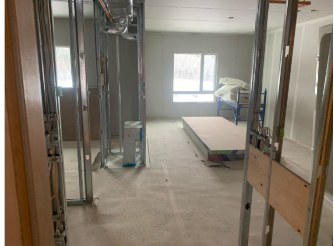
LVL 2 – 1 Bedroom Electrical Rough Ins complete. Backing/Mechanical ongoing.
