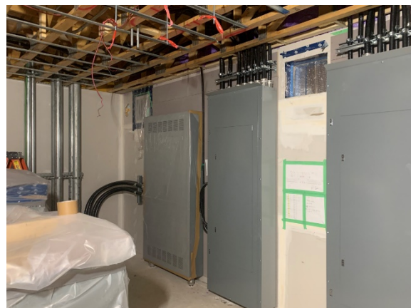
Electrical feeder to building panel tie in complete
