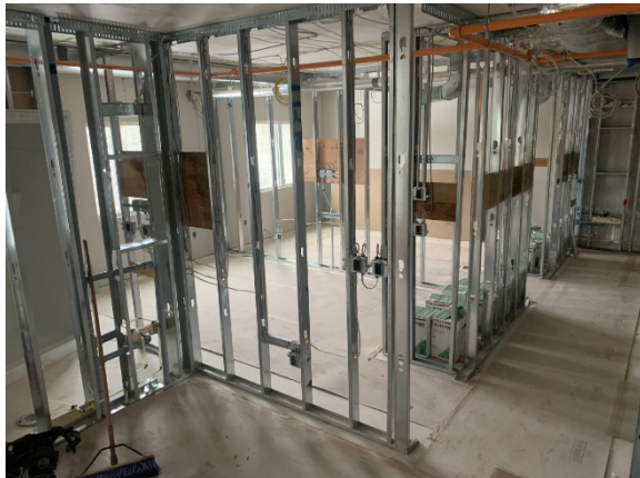
LVL 2 – 3 Bedroom Electrical Rough In complete. Mechanical Rough In and Backing ongoing.
