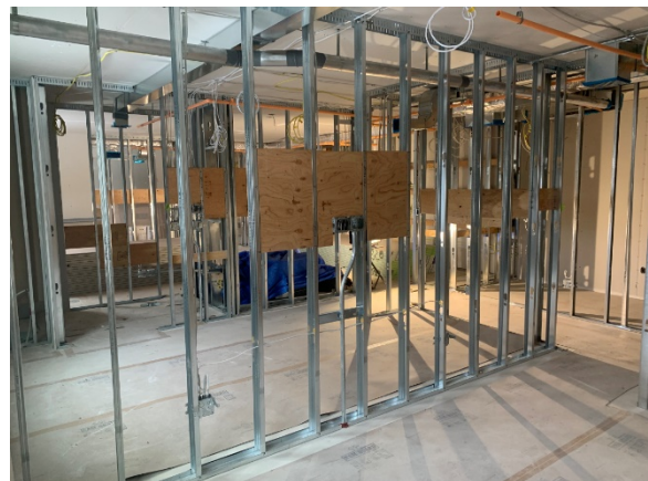
LVL 2 – 3 Bedroom Electrical Rough In complete. Mechanical Rough Ins and Backing ongoing.
