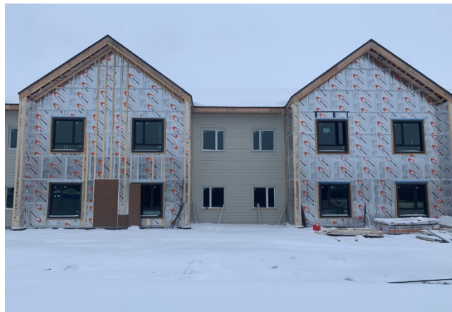
Exterior – North Elevation Fiber Cement progress
