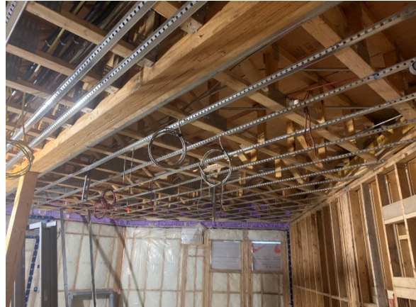
Mechanical Room ceilings prepped for boarding
