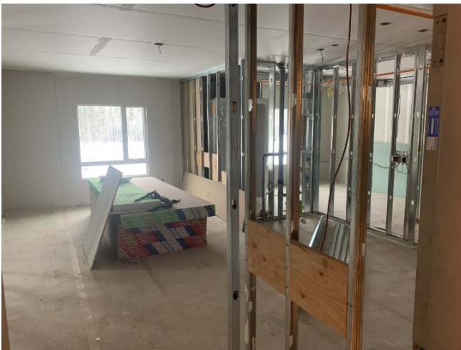
LVL 2 – 2 Bedroom Electrical Rough Ins complete. Backing ongoing. Gypsum board delivered.
