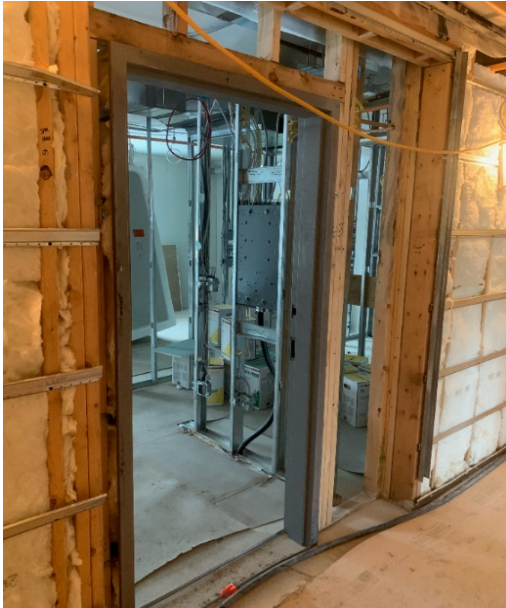
LVL 2 East Wing Hollow Metal Door Frame Install
