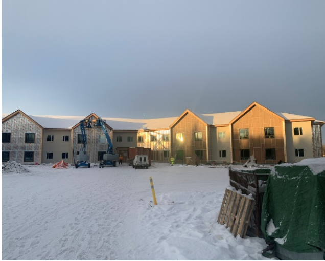
Installation of Fiber Cement Siding
