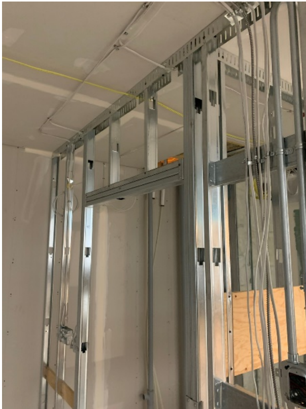
Installation of Heavy Gauge Studs
