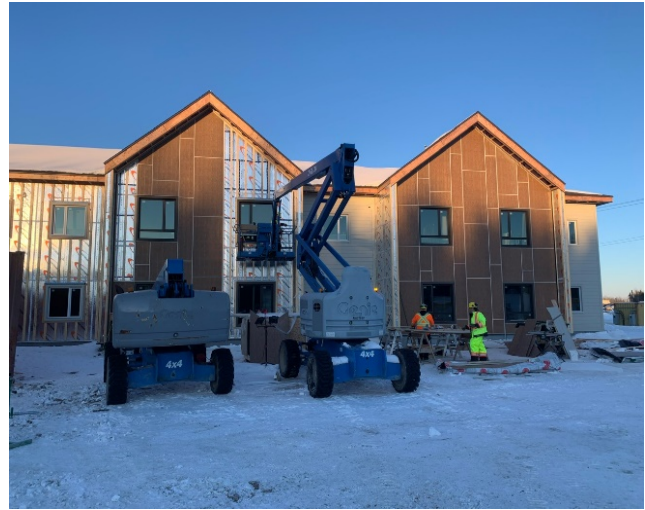
Installation of Fiber Cement Siding
