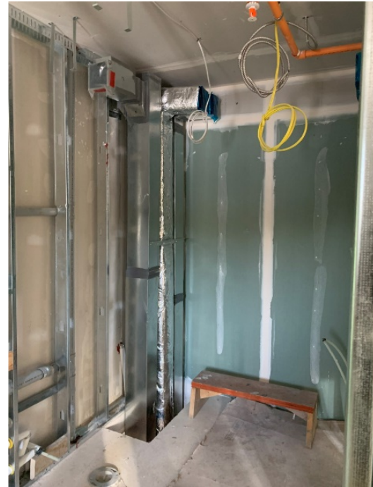
Duct Riser Install
