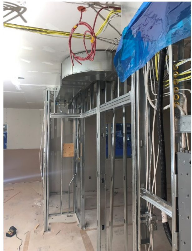
Installation of Heavy Gauge Studs
