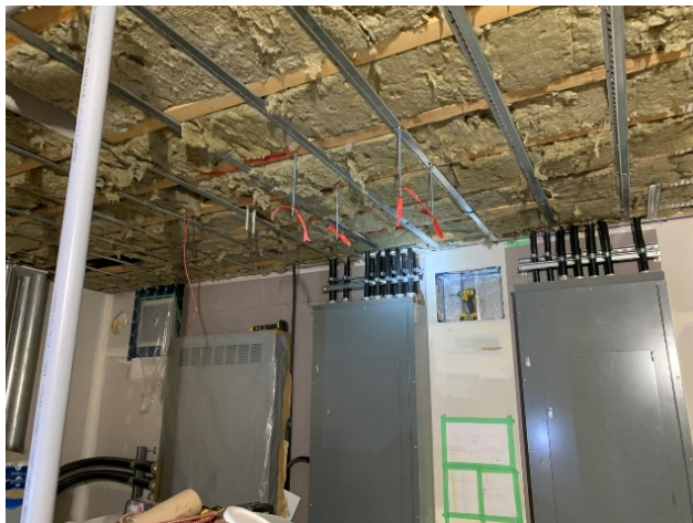
Insulation Above Electrical Room
