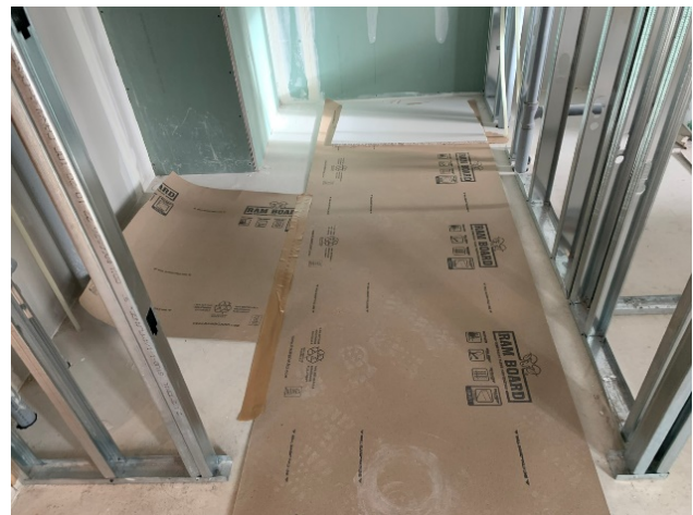
Ram Board Install/Replacement
