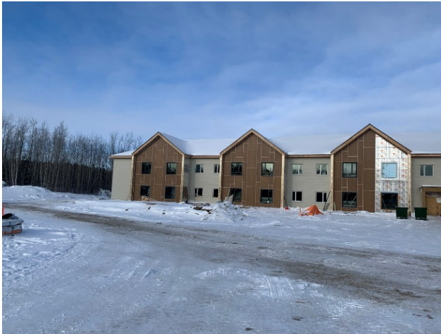
Fibre Cement Siding Install
