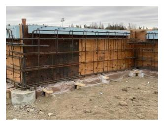
Grade beam formwork with rebar Arshdeep Grewal Dec 13, 2020 8:27 PM
