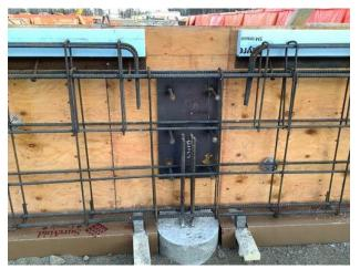
Steel embed in grade beam formwork Arshdeep Grewal Dec 13, 2020 8:15 PM
