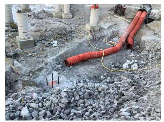
removal of heating unit from poured concrete Wayne Dee Dec 12, 2020 2:08 PM
