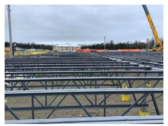
steel joist erection in area A1 Wayne Dee Dec 12, 2020 2:05 PM
