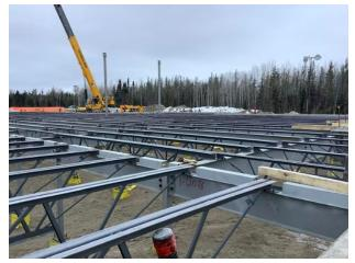
steel joists and beams in area A1 Wayne Dee Dec 12, 2020 2:05 PM
