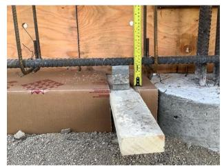
rebar to void spacing confirmation Arshdeep Grewal Dec 13, 2020 8:15 PM
