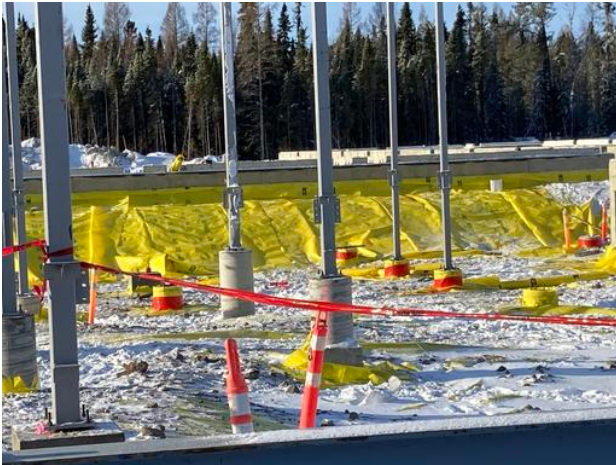
Attaching membrane to Grade beam
