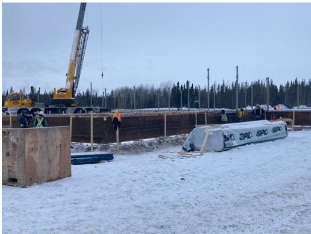
A2- Tying Rebar For Grade Beam Anmol Kang Jan 15, 2021 11:43 AM
