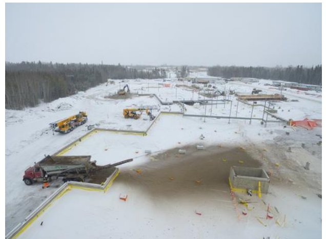
B1- Aerial View of Stone Slinger Spreading Sand
