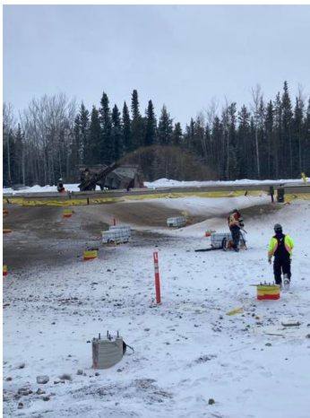
B1- Spreading Sand with Stone Slinger
