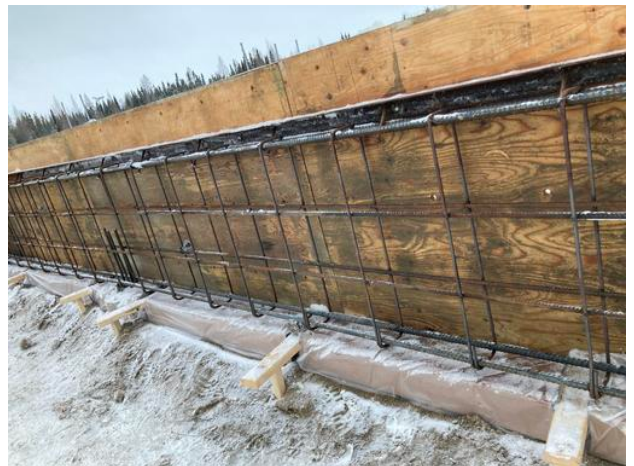
Grade Beam Rebar Closeup
