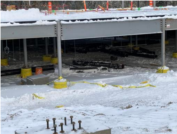
Installation of heating mains under the Qdeck A1
