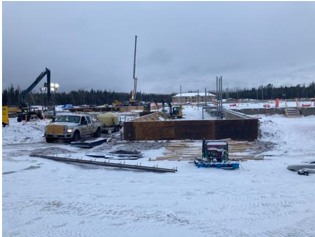
A1- Grade Beam Formwork Anmol Kang Jan 15, 2021 11:43 AM
