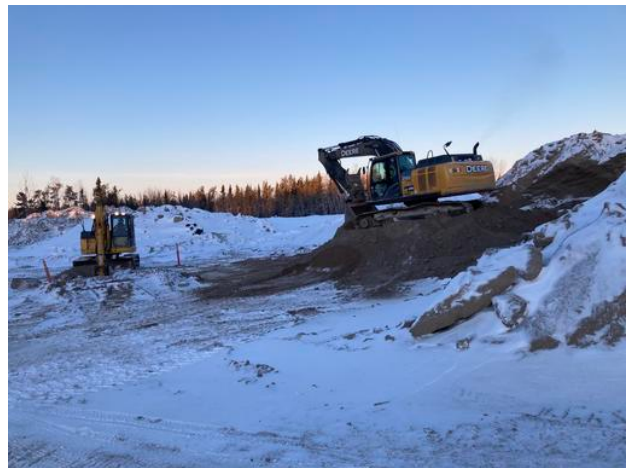
Moving sand for backfill
