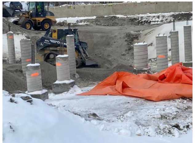
C2- Placing backfill material
