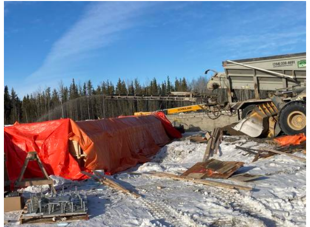
C1- Stone Slinger Spreading Sand
