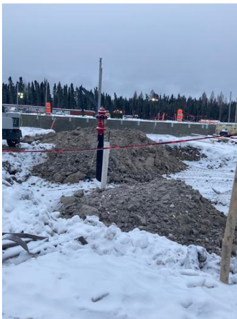
Backfill Sewage and Water Lines Trench
