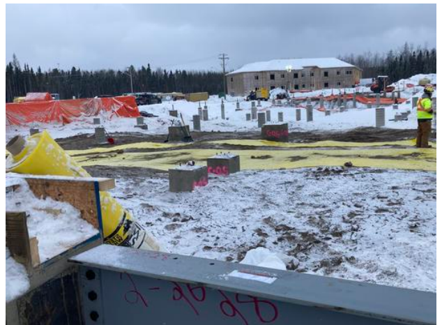
C1- Laying Poly Membrane
