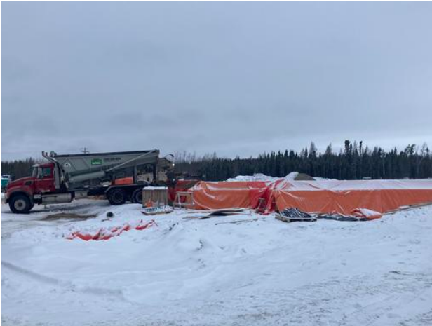
C1- Spreading Sand by Stone Slinger
