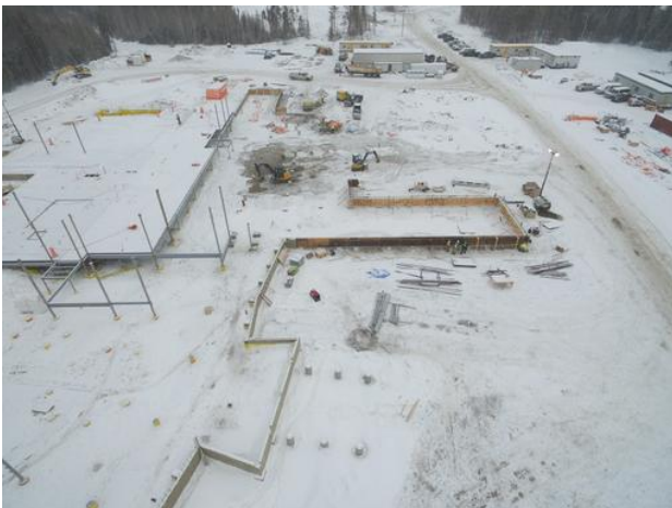
A2- Aerial View of Grade Beam Formwork
