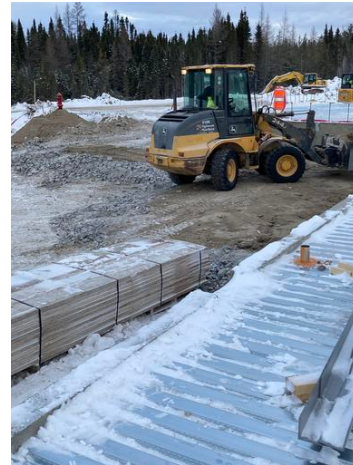
Backfilling near sewage and water connection area
