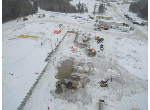
Aerial View of Backfilling Weeping Tiles Trench
