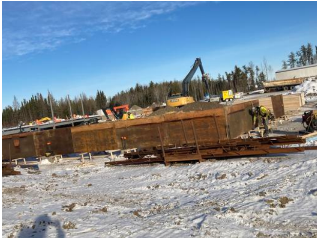
A2- Grade Beam Formwork
