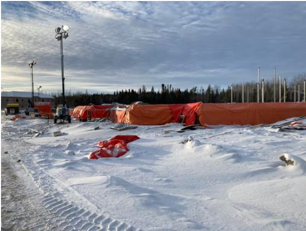
Hoarding over formwork C1
