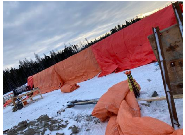
Hoarding over formwork C1
