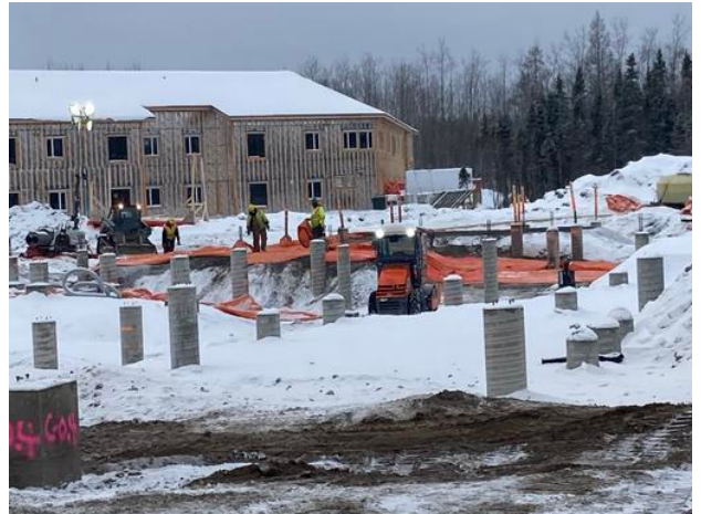
C2- Hoarding & Heating Backfill
