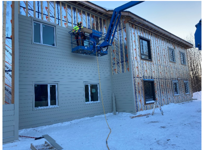
Fibre Cement Siding Install – North
