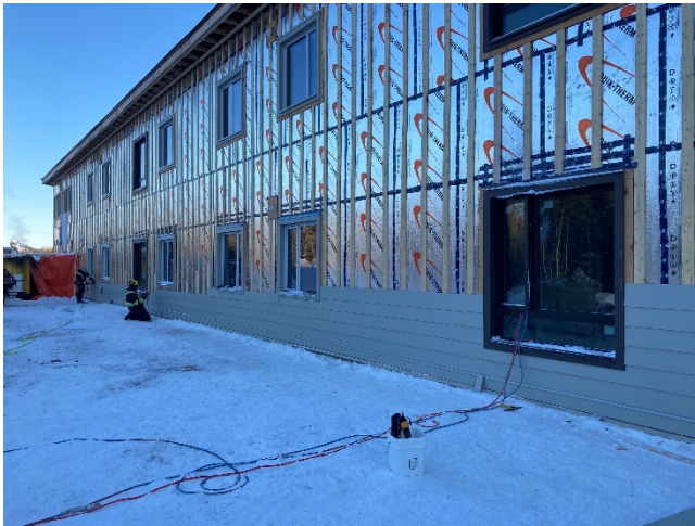
Fibre Cement Siding Install – North
