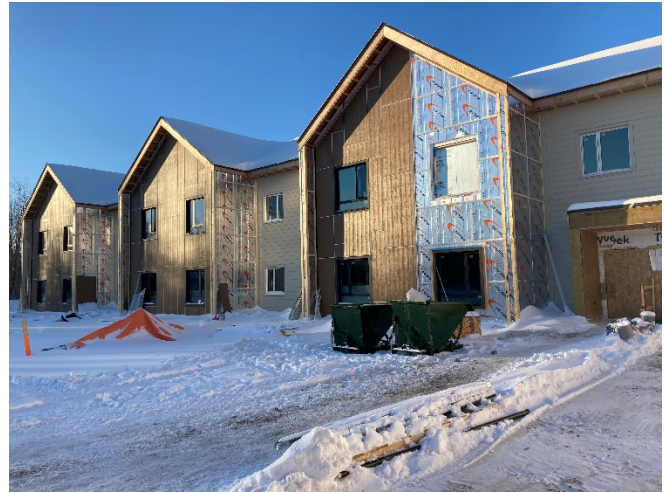
Fibre Cement Siding Install – South
