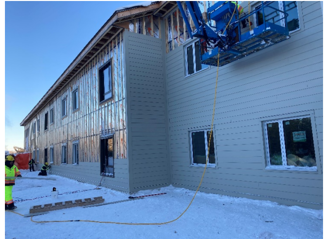
Fibre Cement Siding Install – North
