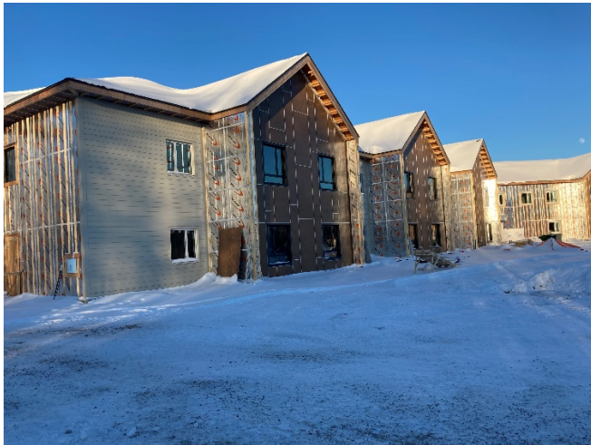
Fibre Cement Siding Install – South
