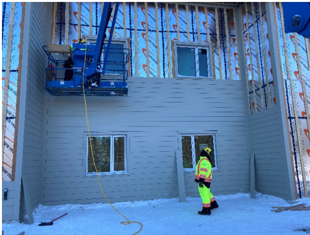
Fibre Cement Siding Install – North
