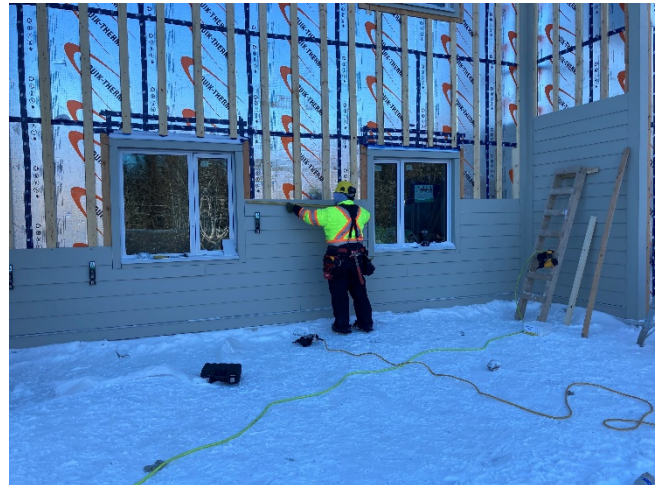
Fibre Cement Siding Install – North
