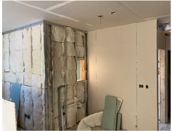
Acoustic Insulation/Gypsum Board Install
