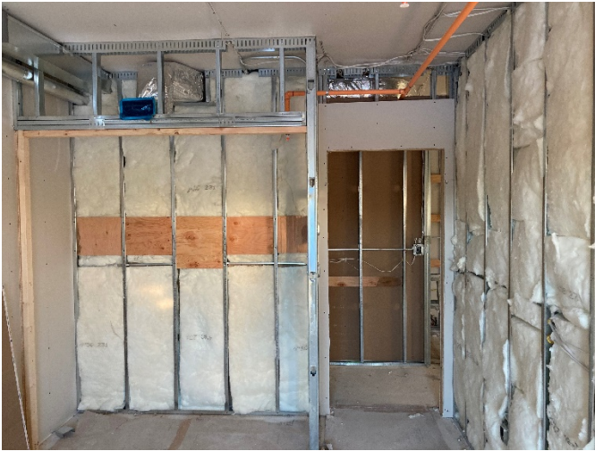
Acoustic Insulation/Gypsum Board Install
