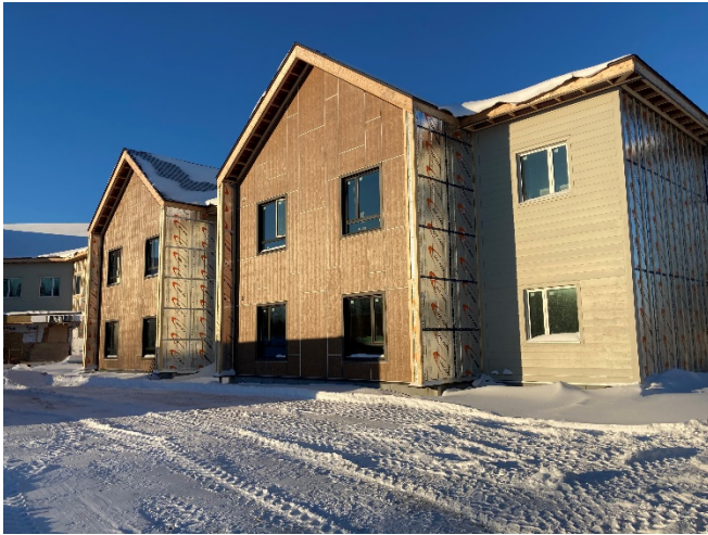
Fibre Cement Siding Install – South
