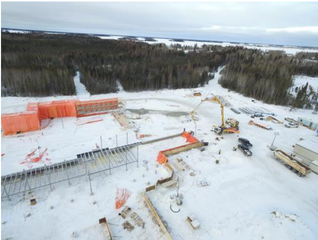
A1- Aerial View of Concrete Pour For Grade Beam
