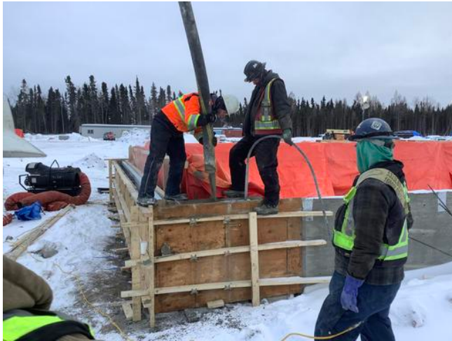
A1- Pouring Concrete For Grade Beam
