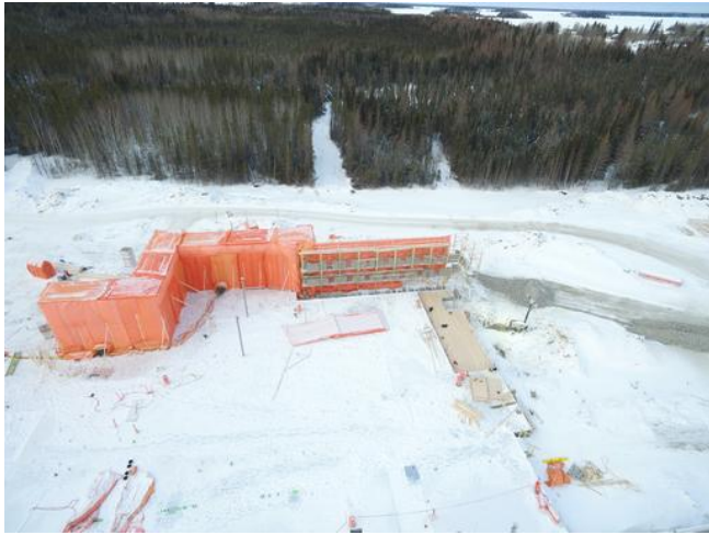
A1- Heating & Hoarding Masonry Wall
