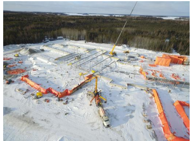
Aerial View - Concrete Pour For Grade Beam (C1)
