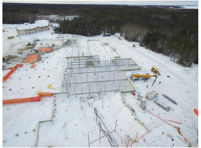
A3/B1 - Aerial View of Steel Erection
