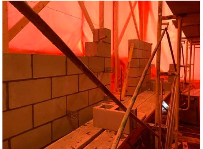
A1- Block Installation For Masonry Wall
