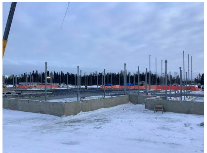
B1- Structural Steel Erection
