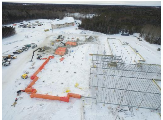
C1- Heating & Hoarding Grade Beam
