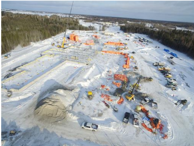
C2- Aerial View of Backfilling Operations
