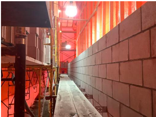
A1- Block Installation For Masonry Wall
