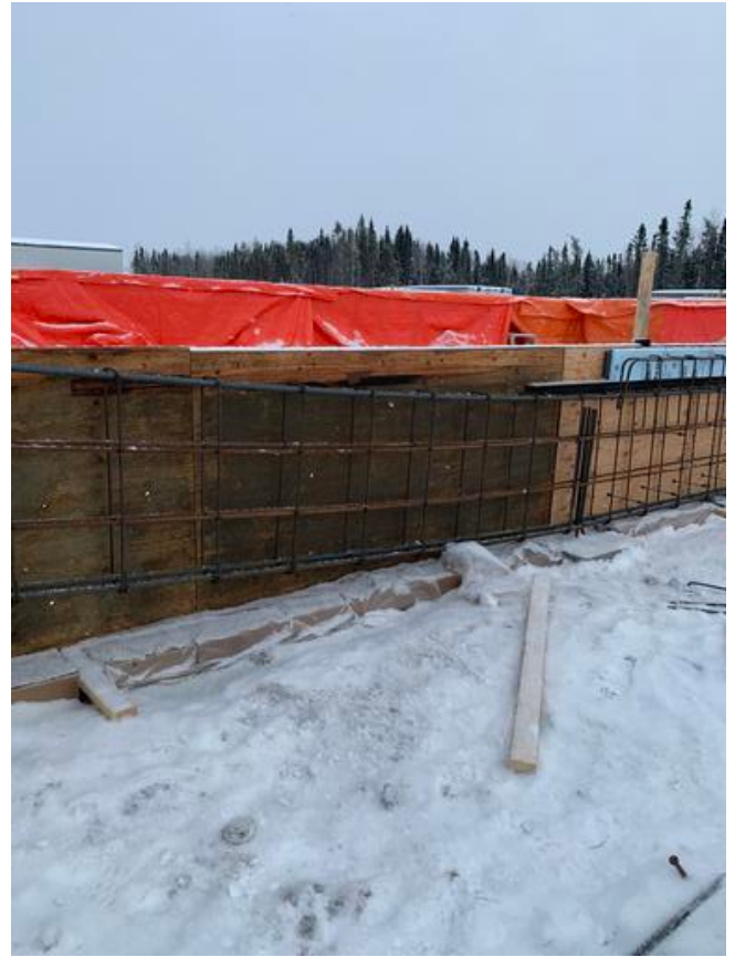
A2- Grade Beam Rebar Arshdeep Grewal Jan 31, 2021 3:34 PM
