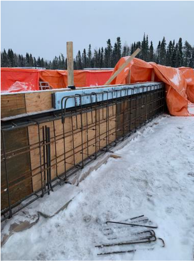
A2- Grade Beam Rebar Arshdeep Grewal Jan 31, 2021 3:34 PM
