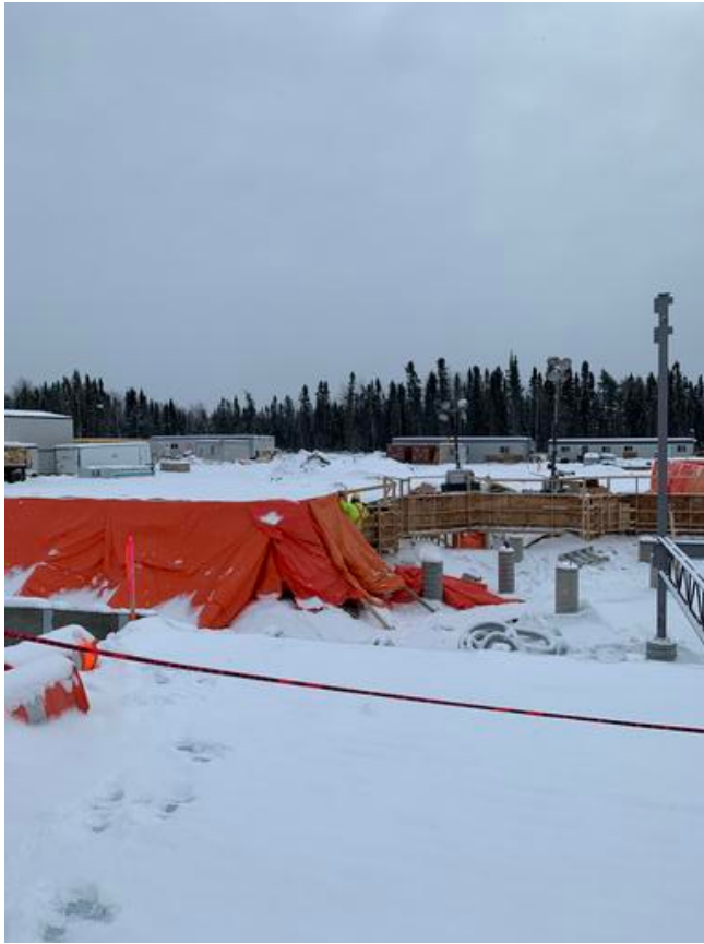
A2- Placing Hoarding Over Grade Beam Arshdeep Grewal Jan 31, 2021 3:34 PM
