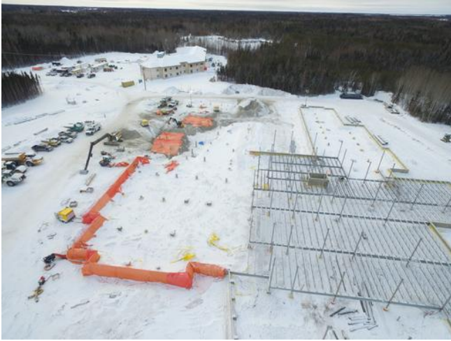
C1- Heating & Hoarding Grade Beam
