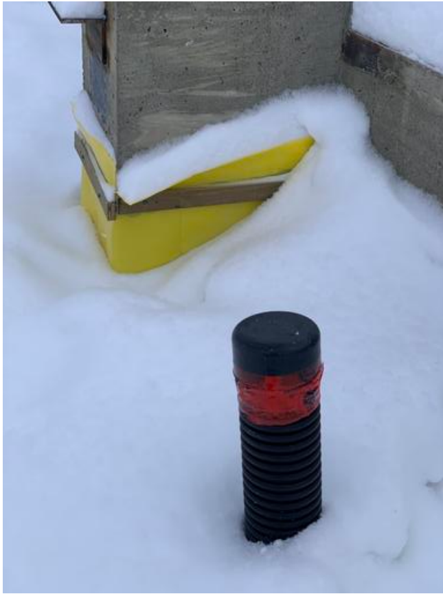
Protecting weeping tile inlets Arshdeep Grewal Jan 31, 2021 3:34 PM
