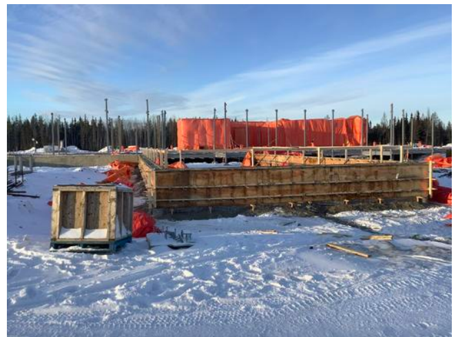
A2- Grade Beam Formwork
