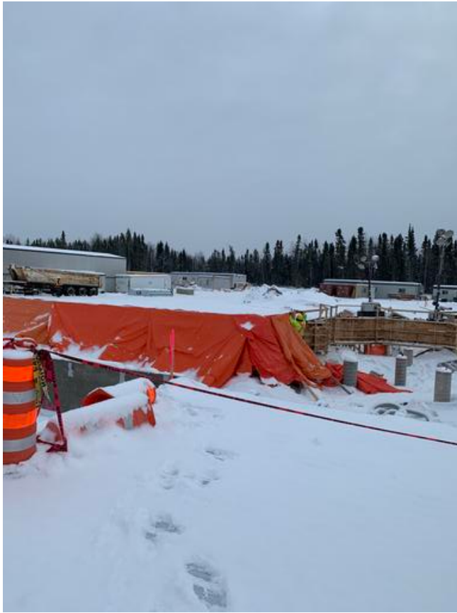
A2- Placing Hoarding Over Grade Beam
