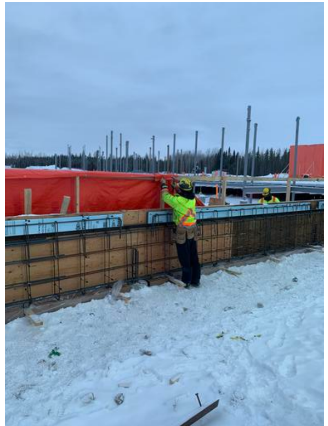
A2- Building hoarding For Grade Beam Arshdeep Grewal Jan 30, 2021 5:35 PM
