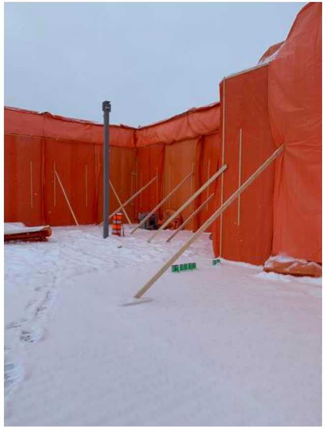
A1- Heating & Hoarding Masonry Wall
