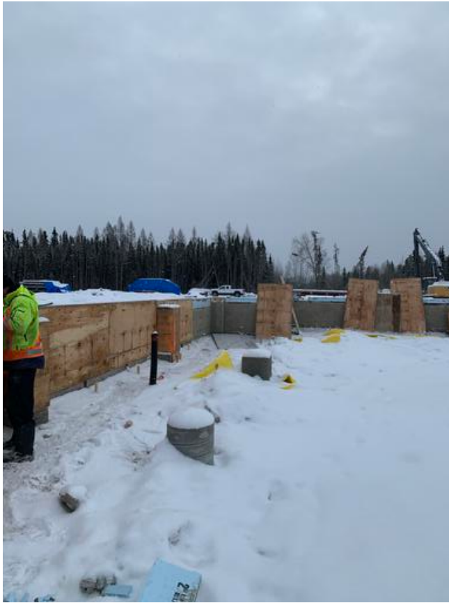
C1- Stripping Formwork From Grade Beam Arshdeep Grewal Jan 31, 2021 3:34 PM
