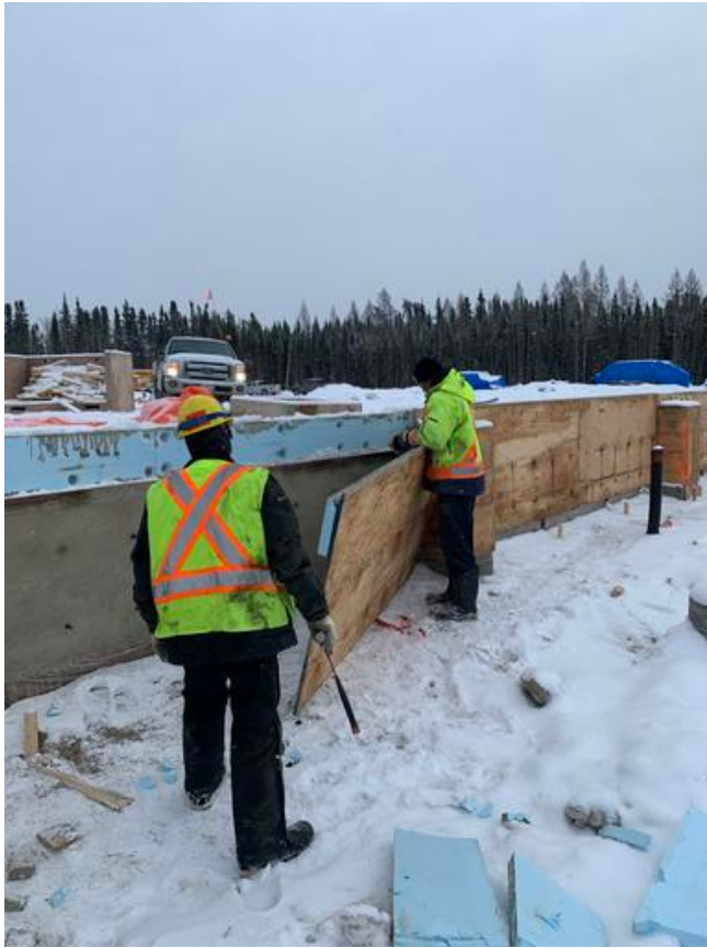
C1- Stripping Formwork From Grade Beam
