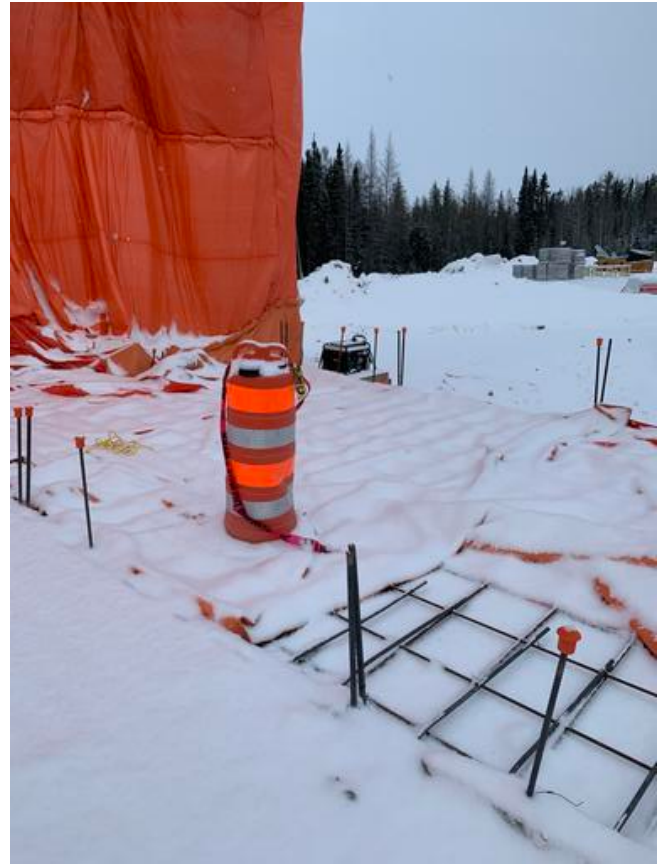
A1- Traps over Structural Slab Arshdeep Grewal Jan 31, 2021 3:34 PM
