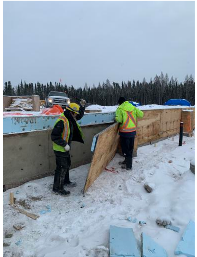
C1- Stripping Formwork From Grade Beam Arshdeep Grewal Jan 31, 2021 3:34 PM
