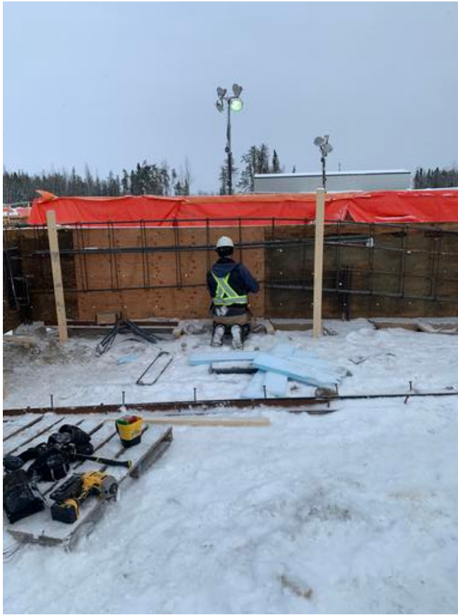
A2- Tying Rebar For Grade Beam Arshdeep Grewal Jan 31, 2021 3:34 PM
