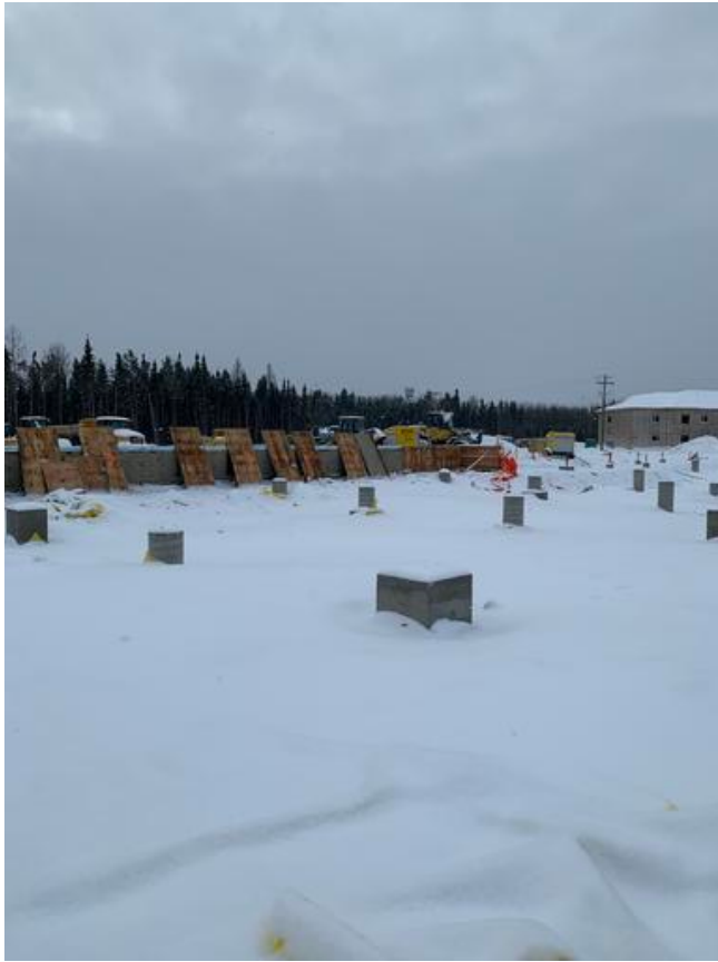
C1- Stripped Formwork From Grade Beam Arshdeep Grewal Jan 31, 2021 3:34 PM
