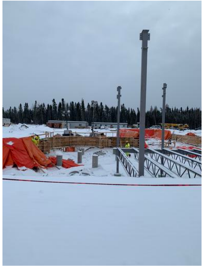
A1- Structural Steel Without Decking
