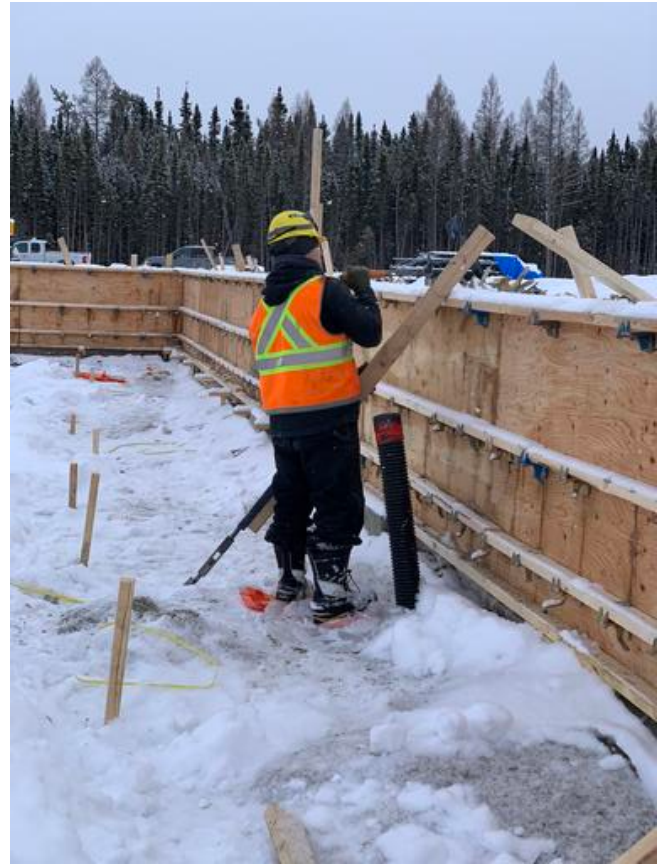
A2- Stripping Formwork From Grade Beam Arshdeep Grewal Jan 31, 2021 3:34 PM
