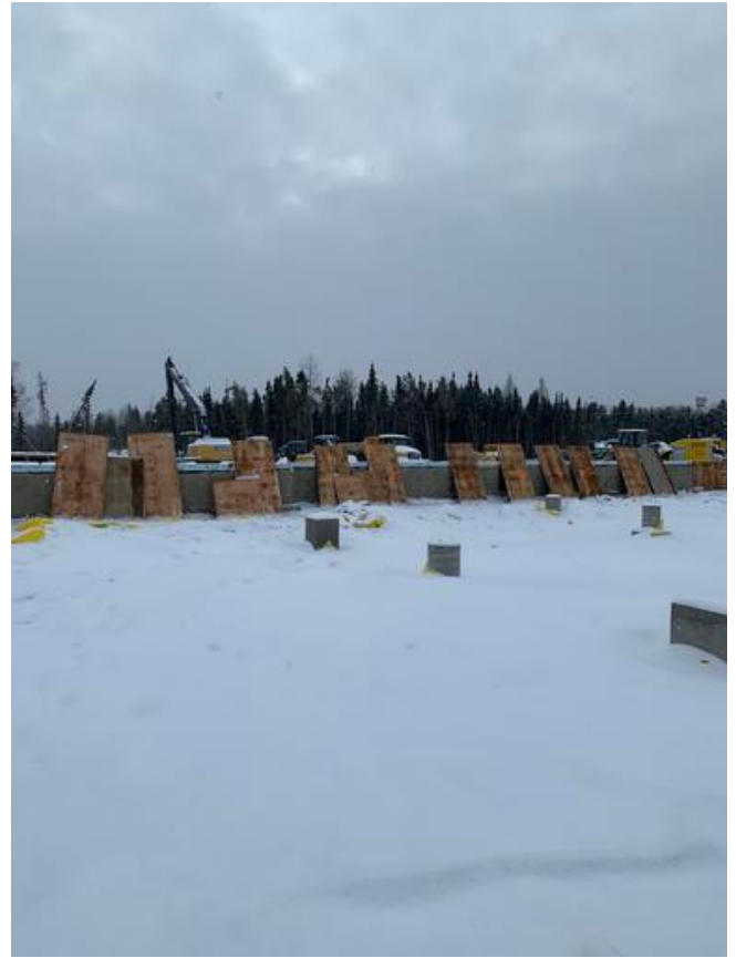
C1- Stripped Formwork From Grade Beam Arshdeep Grewal Jan 31, 2021 3:34 PM
