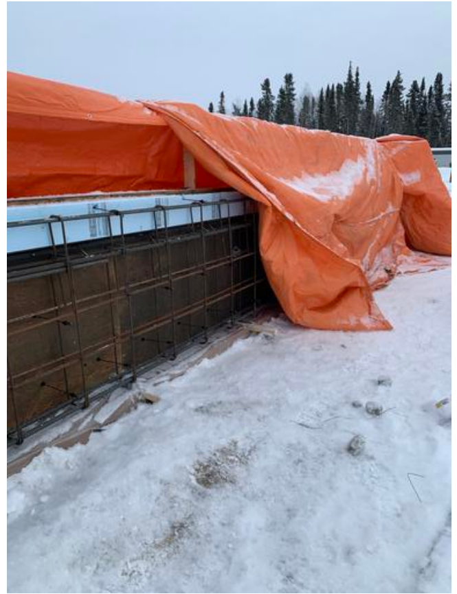
A2- Placing Hoarding Over Grade Beam Arshdeep Grewal Jan 31, 2021 3:34 PM
