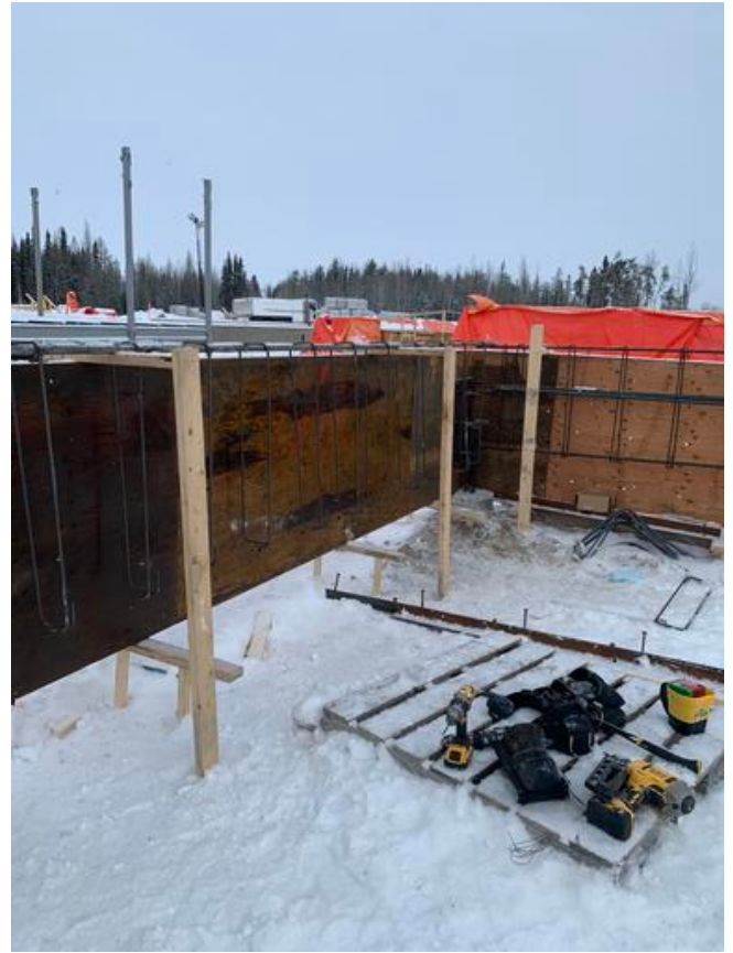
A2- Grade Beam (Formwork & Rebar) Arshdeep Grewal Jan 31, 2021 3:34 PM
