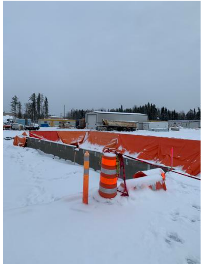
A1- Heating & Hoarding Grade Beam
