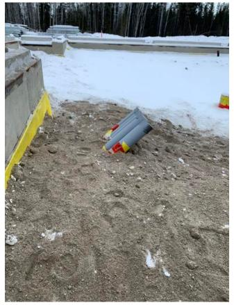
B2- Installed sleeves under Grade Beam Arshdeep Grewal Feb 2, 2021 2:18 PM
