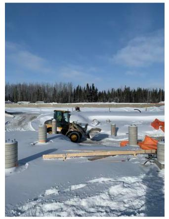
C2- Loader hauling backfill material Arshdeep Grewal Feb 6, 2021 12:42 PM
