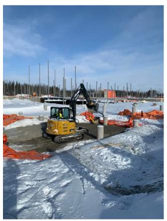
C2- Mini-excavator placing backfill material Arshdeep Grewal Feb 6, 2021 12:42 PM
