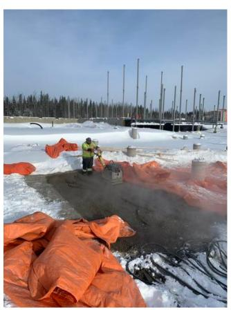
C2- Compacting backfill material Arshdeep Grewal Feb 6, 2021 12:42 PM
