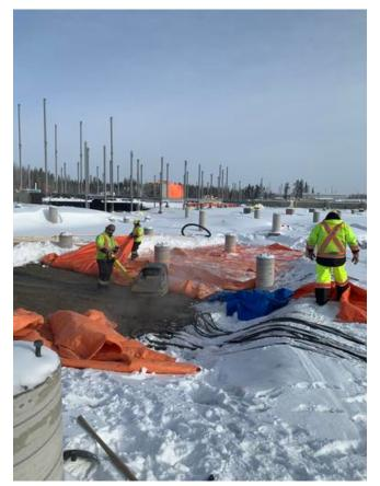
C2- Compacting backfill material Arshdeep Grewal Feb 6, 2021 12:42 PM
