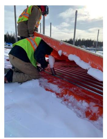
A1- Installation of sleeves in Q-Deck Arshdeep Grewal Feb 6, 2021 12:42 PM
