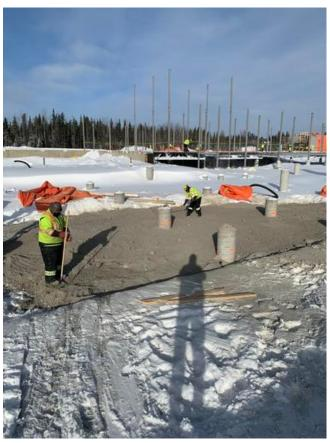
C2- Spreading backfilling material Arshdeep Grewal Feb 6, 2021 12:42 PM
