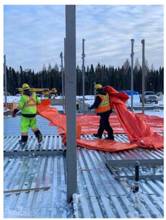
A1- Placing Tarps Over Q-Deck Arshdeep Grewal Feb 1, 2021 4:28 PM
