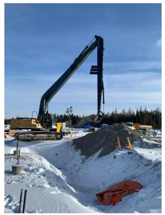
C2- Excavator placing backfill material Arshdeep Grewal Feb 6, 2021 12:42 PM
