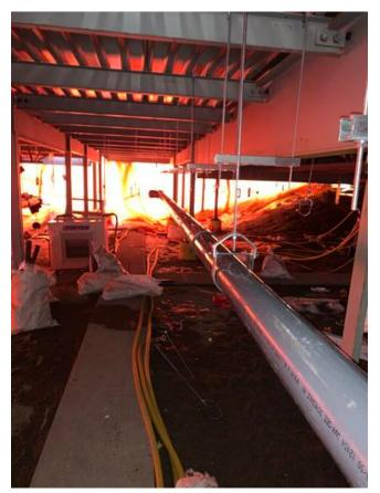
A1- Installing sanitary lines in crawlspace Arshdeep Grewal Feb 5, 2021 10:59 AM
