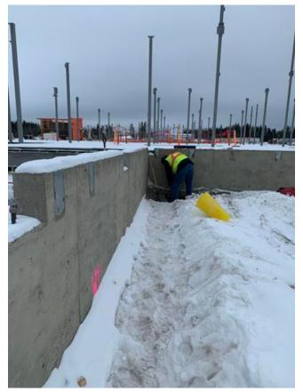
B1- Installing sleeves under Grade Beam Arshdeep Grewal Feb 2, 2021 2:18 PM
