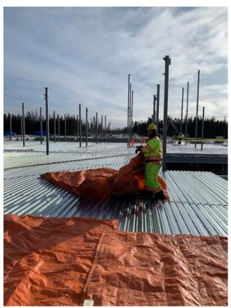
B1- Placing tarps over Q-Deck Arshdeep Grewal Feb 6, 2021 12:42 PM
